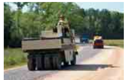
Initial compaction is provided by Ingersoll-Rand pneumatic roller.
