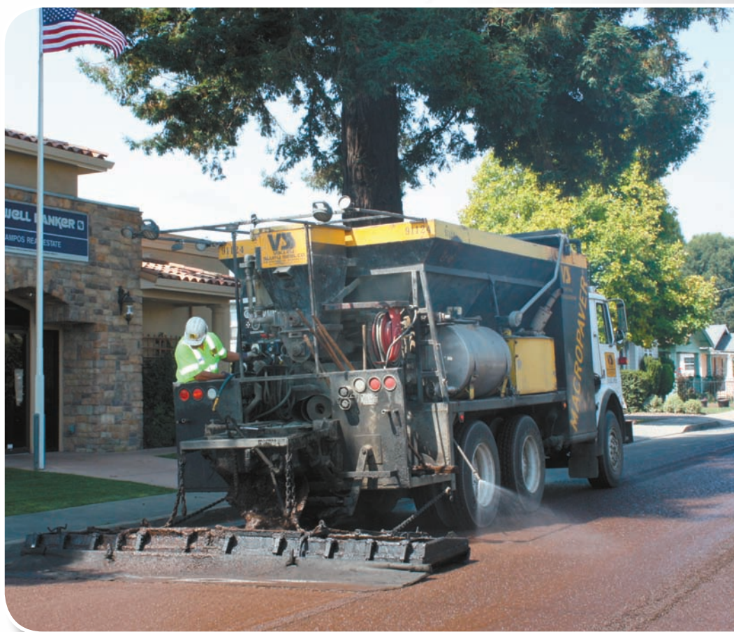
Valley Slurry Seal crew applies micro surfacing on East Lake Street in Watsonville, Calif., as part of City's three-step pavement preservation program.
