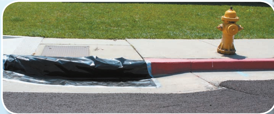
The PW&U department seals catch basins before pavement preservation treatments to prevent contamination of watercourses.
