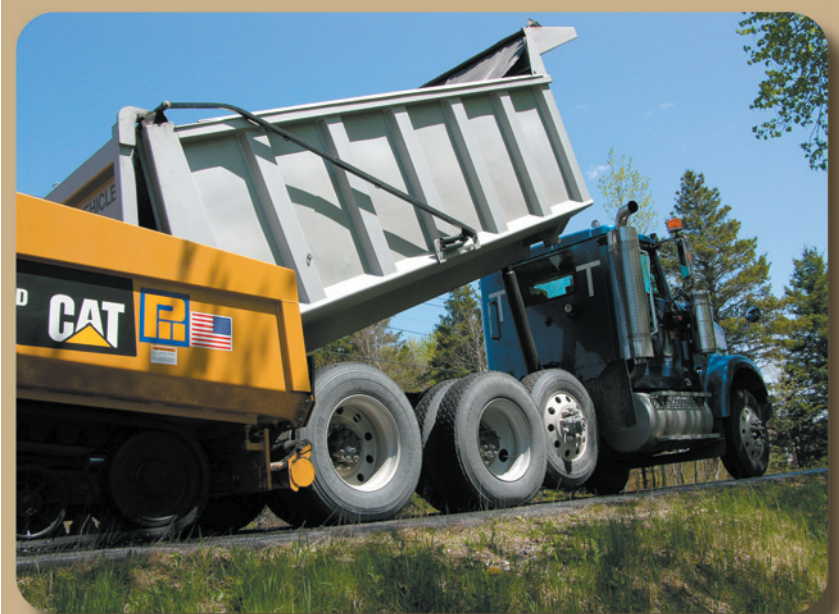
Top: Pike Industries employs a CAT 1055D with a Carlson IV screed to place a 3/4- to 1-inch overlay on Route 114 in Norton, Averill and Canaan.
