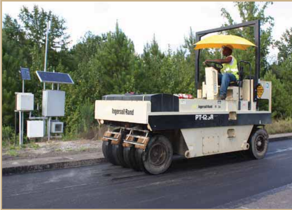
Ingersoll Rand roller passes solar-powered tower that collects information from instruments embedded in pavement and transmits data to research lab.
