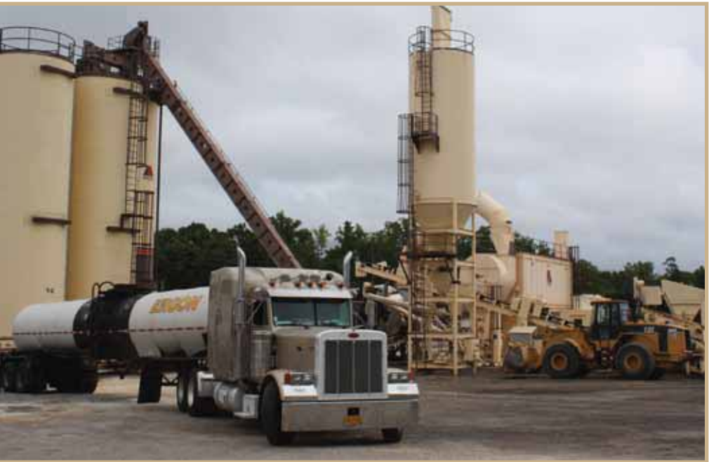
Truck containing binder from Ergon Asphalt & Emulsions hooks up directly to East Alabama’s Astec hot mix plant.
