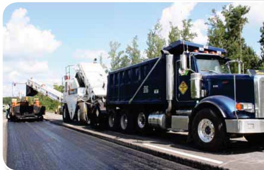
East Alabama Paving's ROADTEC Shuttle Buggy feeds hot mix asphalt containing HiMA binder to Blow Knox paver during NCAT Test Track repair.
