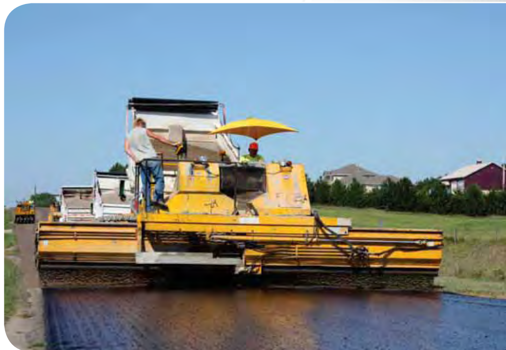
Sta-bilt Construction's Etnyre chip spreader broadcasts stone over asphalt emulsion during chip seal of a Madison County, Neb. road.
