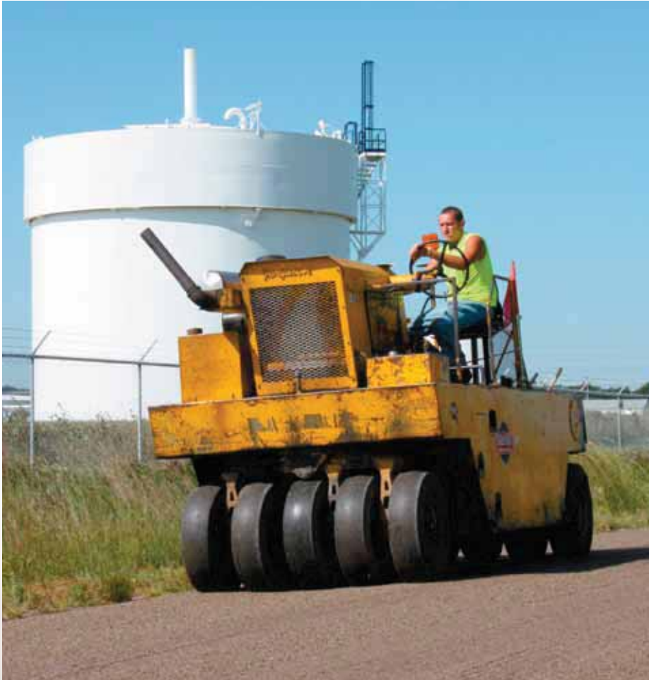
Stone chips are embedded in asphalt emulsion by one of two Ferguson pneumatic rollers used for the project.
