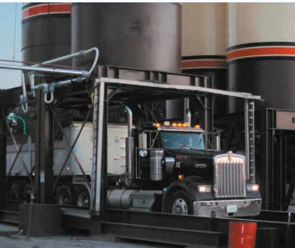
As day fades into dusk, a Kenworth tractor/trailer picks up first load of hot asphalt mix.
