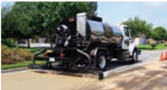
Rejuvenator is placed on Travis County, Tex., streets; the distinctive color disappears when the emulsion 'breaks.'
