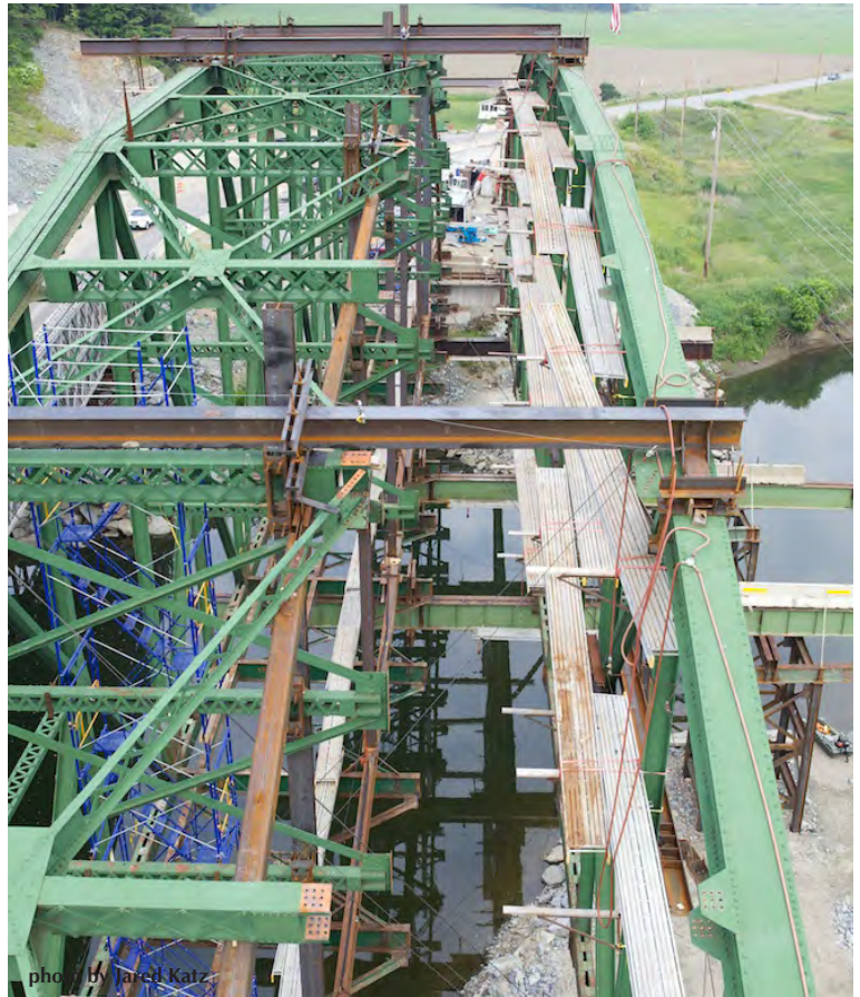
The day after: truss has been moved and the bridge is now 12.5 feet wider.
