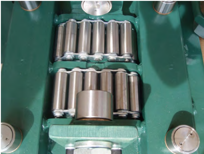
Rollers specially made to fit under the truss allowed the truss to glide when pushed.
