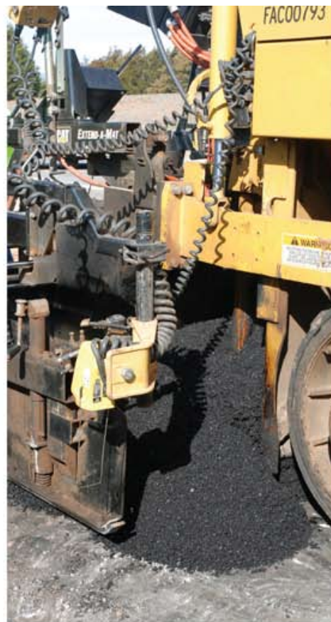
The HiMA mix containing Kraton D0243, a new SBS modifier, is fed under the screed to lay a durable asphalt pavement with a 30 percent reduced pavement depth, which saves money for the Oklahoma DOT.
