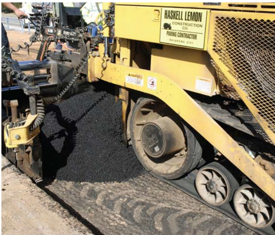
The HiMA mix containing Kraton D0243, a new SBS modifier, is fed under the screed to lay a durable asphalt pavement with a 30 percent reduced pavement depth, which saves money for the Oklahoma DOT.
