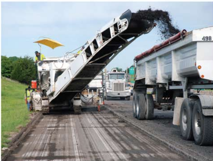
Haskell Lemon's milling crew cold-mills the shoulder of I-40 in advance of HiMA paving.
