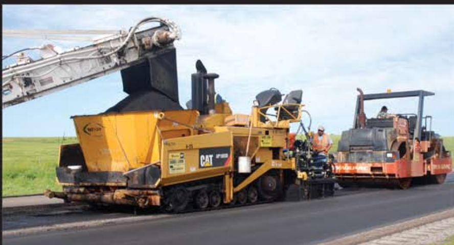
The Haskell Lemon crew hauled the Kraton™ D0243 HiMA mix to a Roadtec Shuttle Buggy, which delivered it in a smooth, steady flow to a hopper insert in a Cat AP1055B paver. The Dynapac double drum roller served in the breakdown position.
