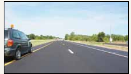
Recently micro surfaced segment of MnROAD’s 3.5-mile mainline test section that periodically carries average daily traffic of 28,000 vehicles from I-94.
