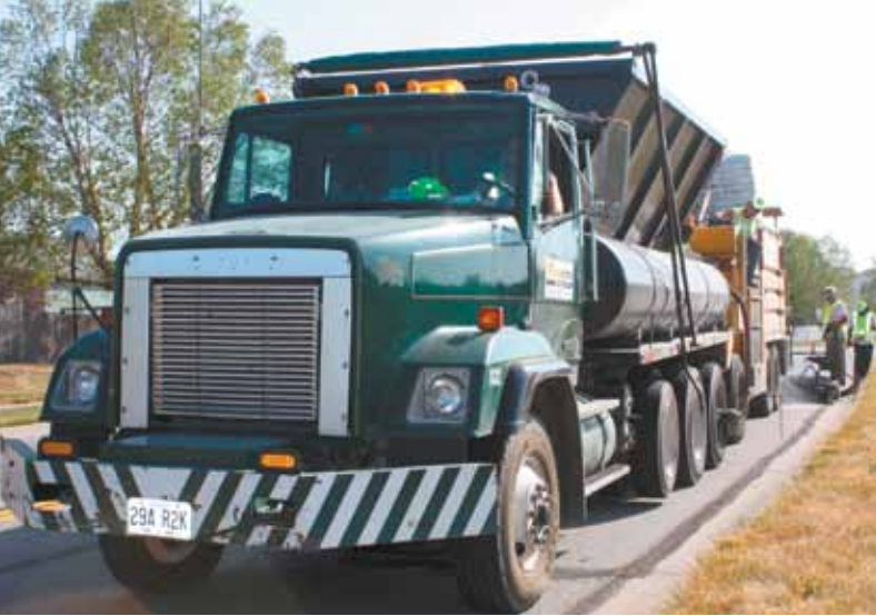
A Freightliner “nurse” truck delivers raw materials to micro surfacing machine.
