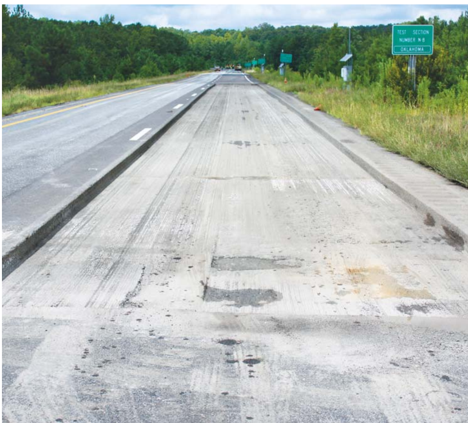
On Aug. 17, 2010, crews removed the top 5 1/4 in. of existing N8 pavement and replaced this with HiMA mix. Truck traffic resumed, and NCAT continued collecting data.
