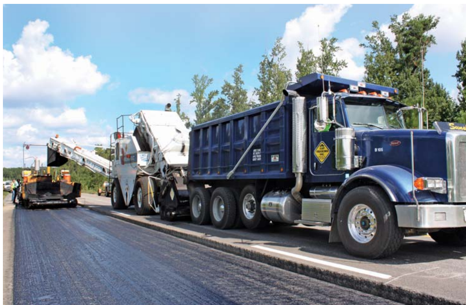
NCAT's 2009-11 research cycle began in August 2009 with the reconstruction of 17 test sections. One of the sections, North 7 (N7), incorporates HiMA technology developed by the sponsor, Houston-based Kraton Performance Polymers.
