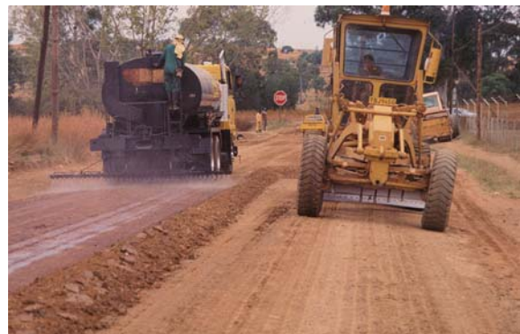
Figure 14. Photo. Mix-in treatment.
