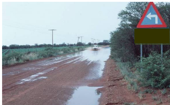
Figure 66. Photo. Road below natural ground level.
