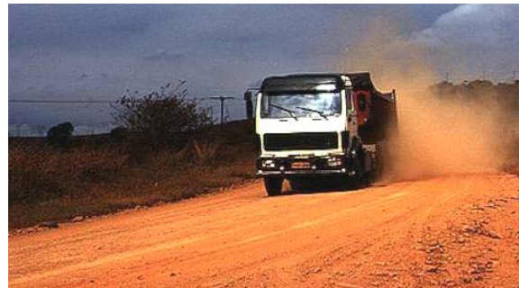
Figure 90. Photo. Road before treatment.
