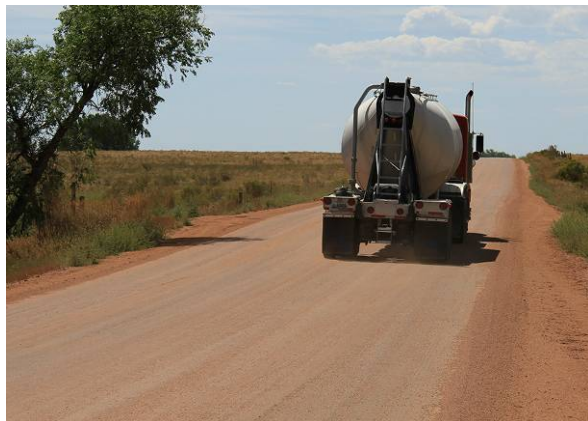
Figure 82. Photo. No dust. (1 on a scale of 1-5).
