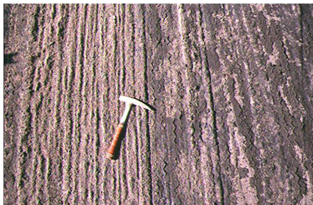
Figure 71. Photo. Poor penetration without pre-wetting.
