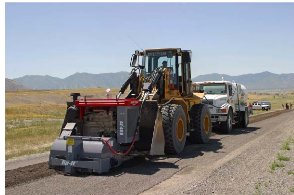
Figure 76. Photo. Equipment-mounted recycler.
