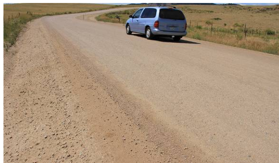
Figure 21. Photo. Road with good drainage.
