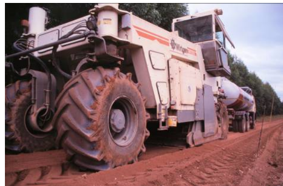
Figure 77. Photo. Full-depth recycler.
