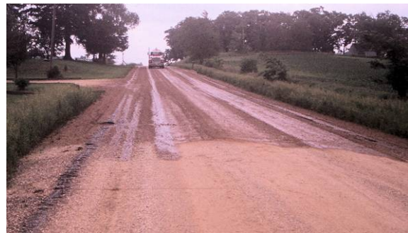
Figure 29. Photo. Lignosulfonate road.
