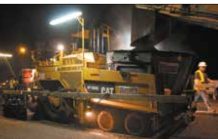
Material transfer vehicle loads HiMA intermediate or binder course into paver.
