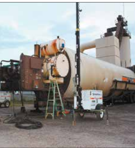
Kraton D0243 HiMA polymer modifier liquid binder from Ergon Asphalt & Emulsions is loaded into Heatec portable tank at APAC Midsouth drum plant in Troy.
