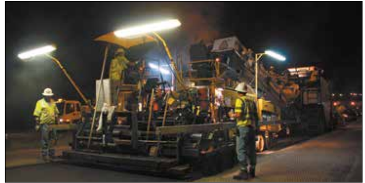
CAT AP-1000D asphalt paver places HiMA intermediate or binder course on U.S. 231 in Troy, Alabama.
