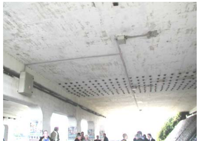
Figure 7.11. In-situ measurements of humidity in concrete. A. Wooden-stick method. B-C. Portable humidity probes. D. Automatic in-situ monitoring of temperature, humidity and expansion (vibrating wire) in a bridge deck affected by ASR (Siemes and Gulikers 2000).
