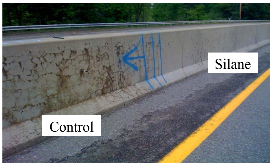
Figure 8.10. Reduction in Cracking of Highway Barriers in Massachusetts, after Application of Silane (FHWA Project DTFH61-06-D-00035)
