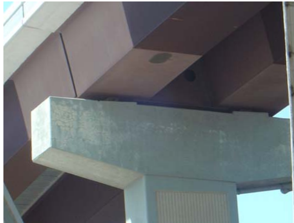
Figure 8.3. Photograph of bridge in Houston, Texas, illustrating effects of moisture availability on ASR-induced expansion and cracking. Only the exposed face of the bent cap (left side of photo) shows visual cracking, whereas the portions of the bent cap protected by the bridge deck show very little cracking.
