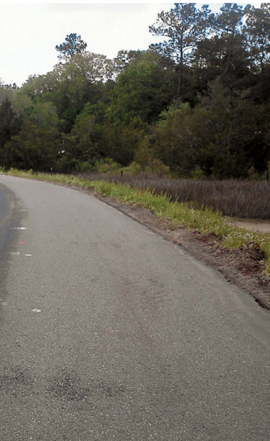
In May 2013, the county completed a test section utilizing Tire Rubber Modified Surface Seal
