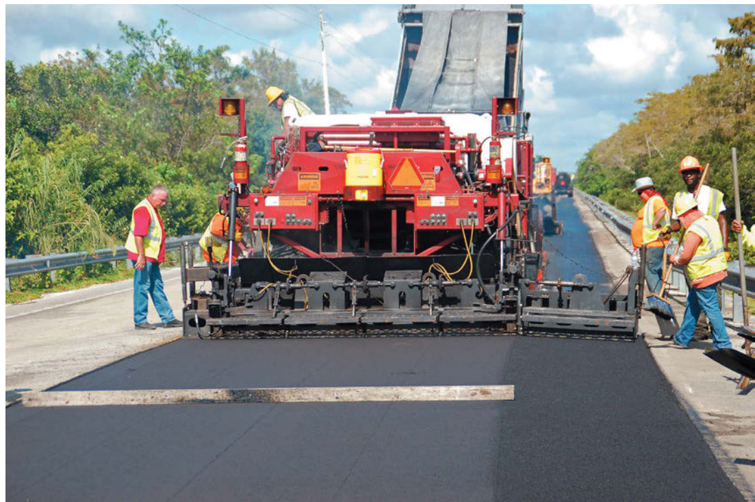
At eastern boundary of Big Cypress National Preserve in far south Florida, repaver begins recycling/repaving of 12-ft. driving lane and 4-ft. repaving of shoulder without recycling
