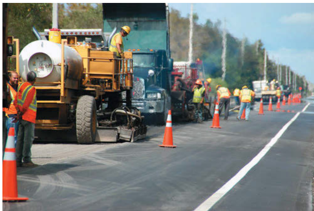
On U.S. 41 Tamiami Trail, hot in-place repaving train includes, from left, mobile preheater, truck delivering hot mix asphalt into mobile recycling unit, and compactors at rear
