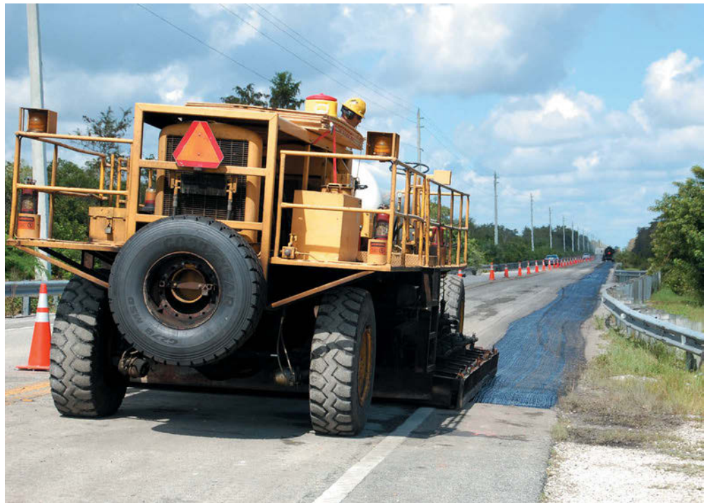
As tack coat is applied to shoulder only in advance of overlay, preheater unit begins movement down driving lane of U.S. 41 in advance of repaver
