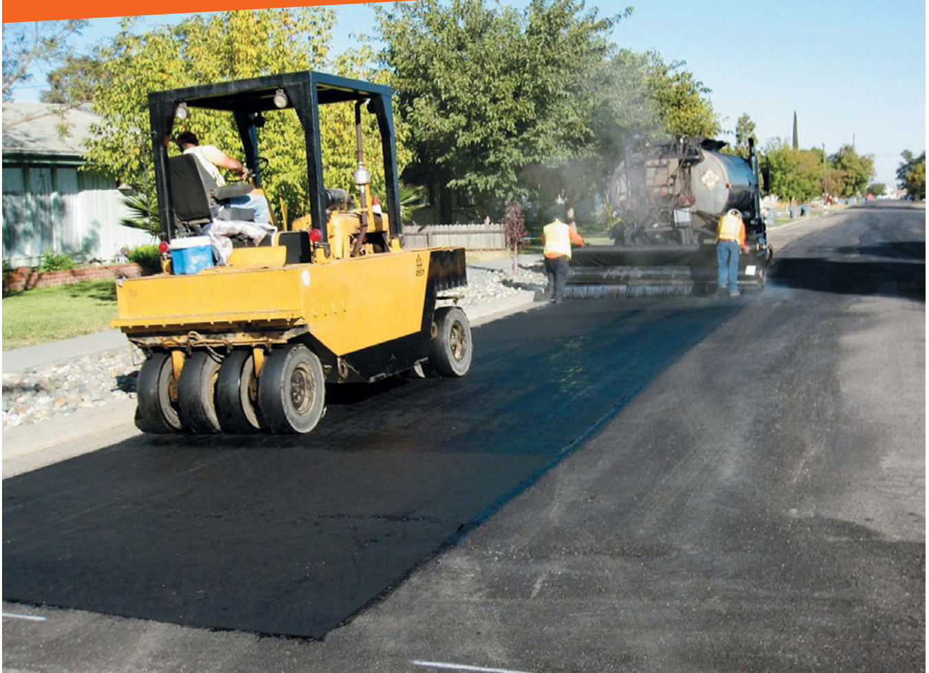
Delta places a 4.1 oz. pavement fabric into a hot oil binder, followed by pneumatic rolling
