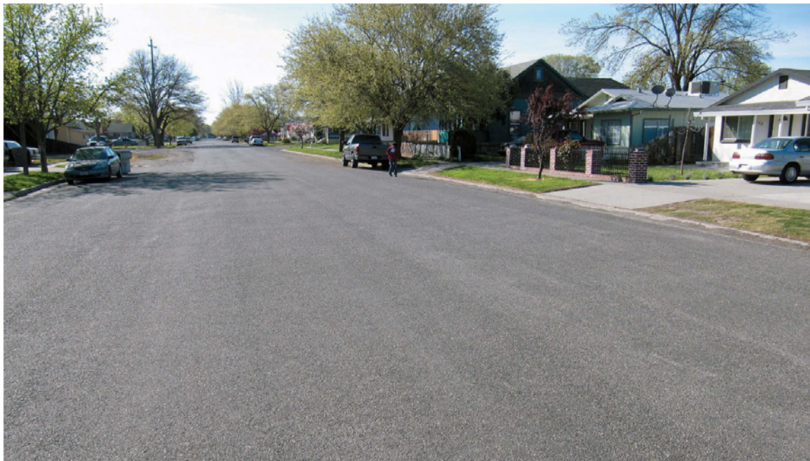
After five years, pavement is intact (compare to same location in photo Page 19)
