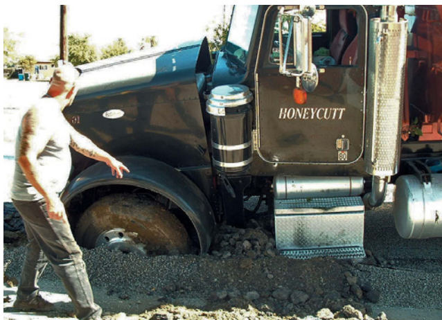
Subgrade in Williams so saturated that trucks could not negotiate streets
