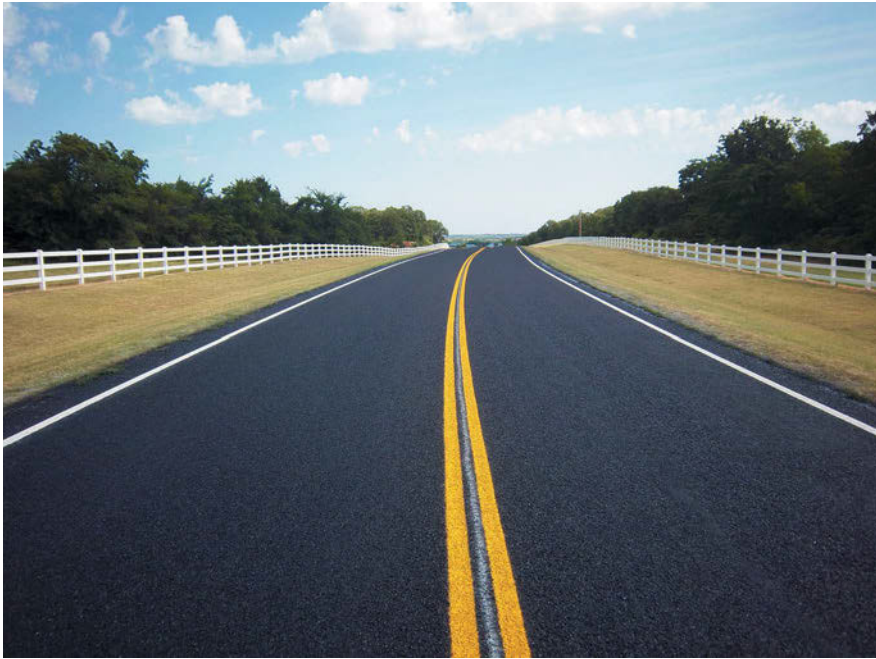
Final product: crack seal, chip seal, and a double fog seal were used to repair this pavement leading to the Chickasaw Children's Village in Kingston, Okla.
