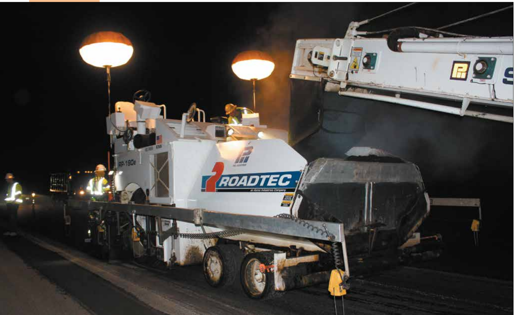
A material transfer vehicle feeds highly modified asphalt mix to Pike Industries' paver during NHDOT's innovative Highways for Life resurfacing of NH101 in Auburn.
