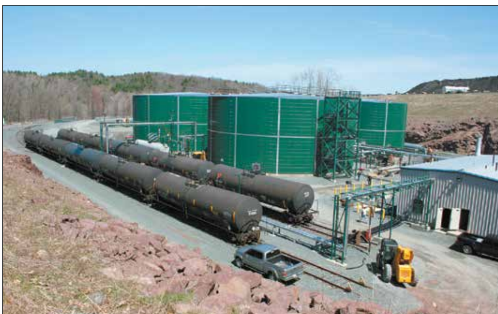
Railroad cars deliver neat asphalt binder to All States Materials Group's Deerfield, Mass., facility for blending with Kraton's D0243 polymer to produce HiMA binder.
