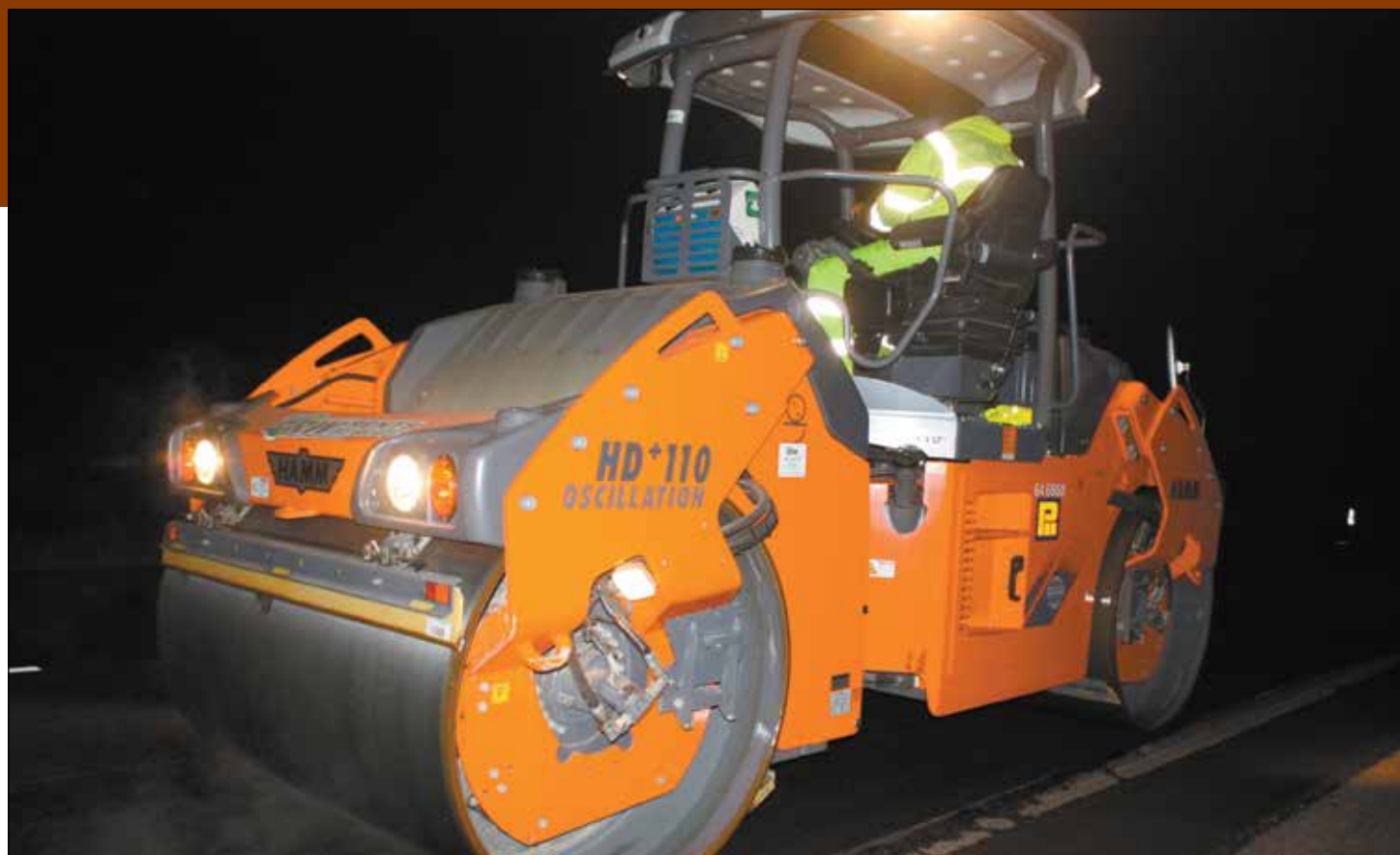
A HAMM HD-110 Compactor is employed as finish roller for wearing course
