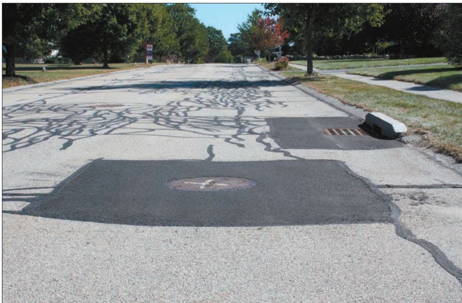
Alligator cracks around manholes and other structures were removed by Felix A Marino Co. using infrared machines and Mari-Mix high-performance patching material
