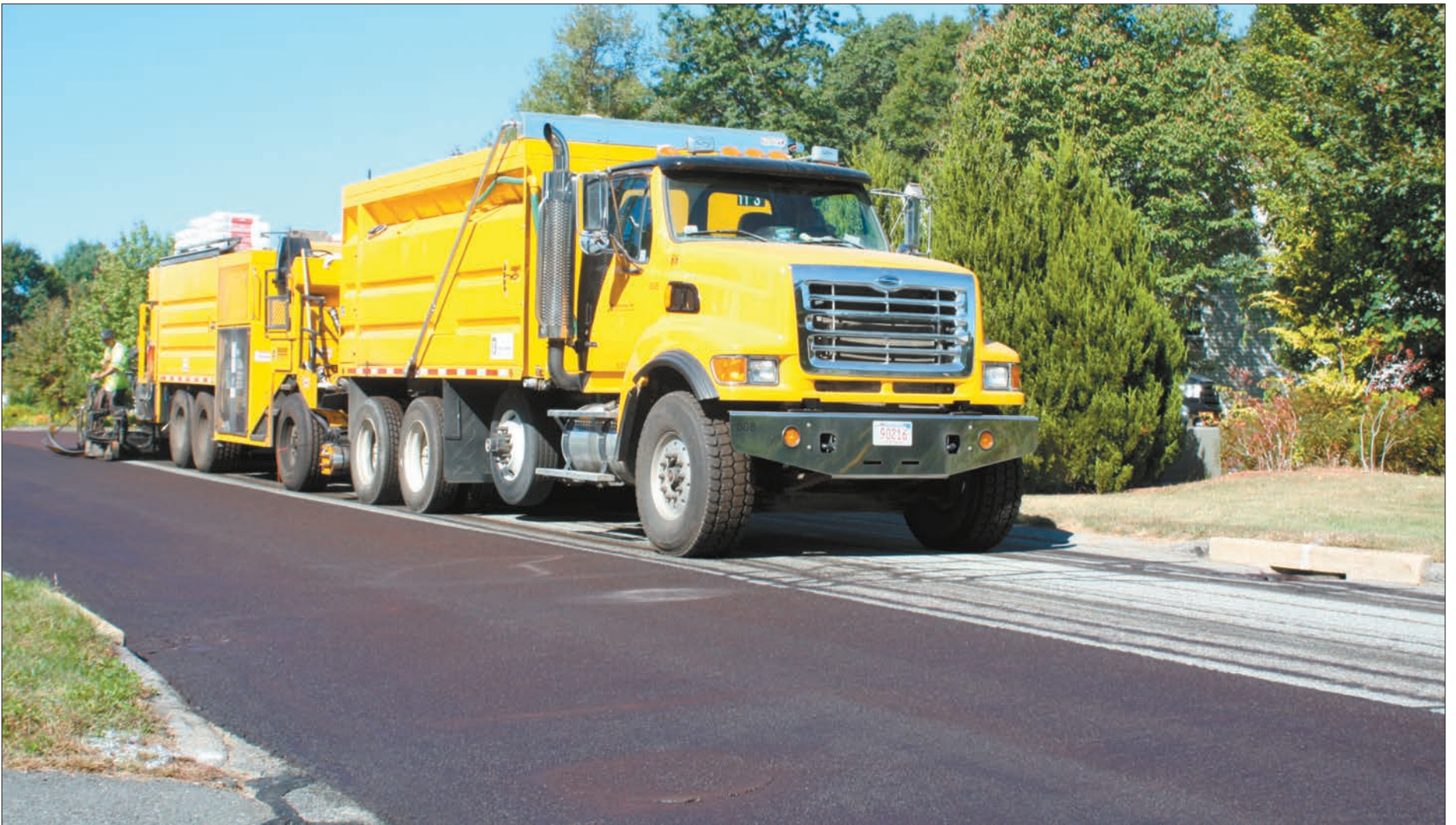
A Sterling nurse truck feeds materials to Bergkamp paver as town's first micro surfacing takes place
