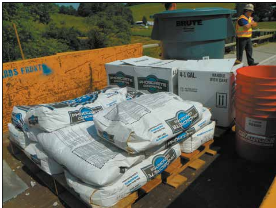
Pallet of magnesium-alumina-aggregate dry powder and containers of mono-aluminum-liquid phosphate activator are stored on trailer till needed for job-site mixing.
