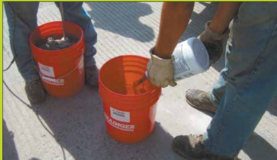
While one 5 gallon pail of powder and liquid activator are mixed with auger, a second pail receives activator for second batch.
