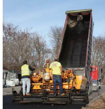
Cooper Bros. Paving first applied a levelling course of HMA over the site then followed this with the placement of the 2-inch top course in a single lift using a LeeBoy 8500 paver.
