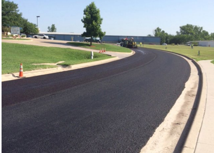
Figure 2. Photographic illustration of a micro surfacing layer
