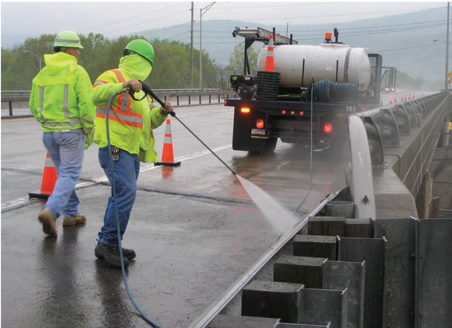
PennDOT workers power wash a bridge structure. Keeping the expansion areas and joints of bridges free of debris and salt accumulation from winter services is a critical maintenance function.
