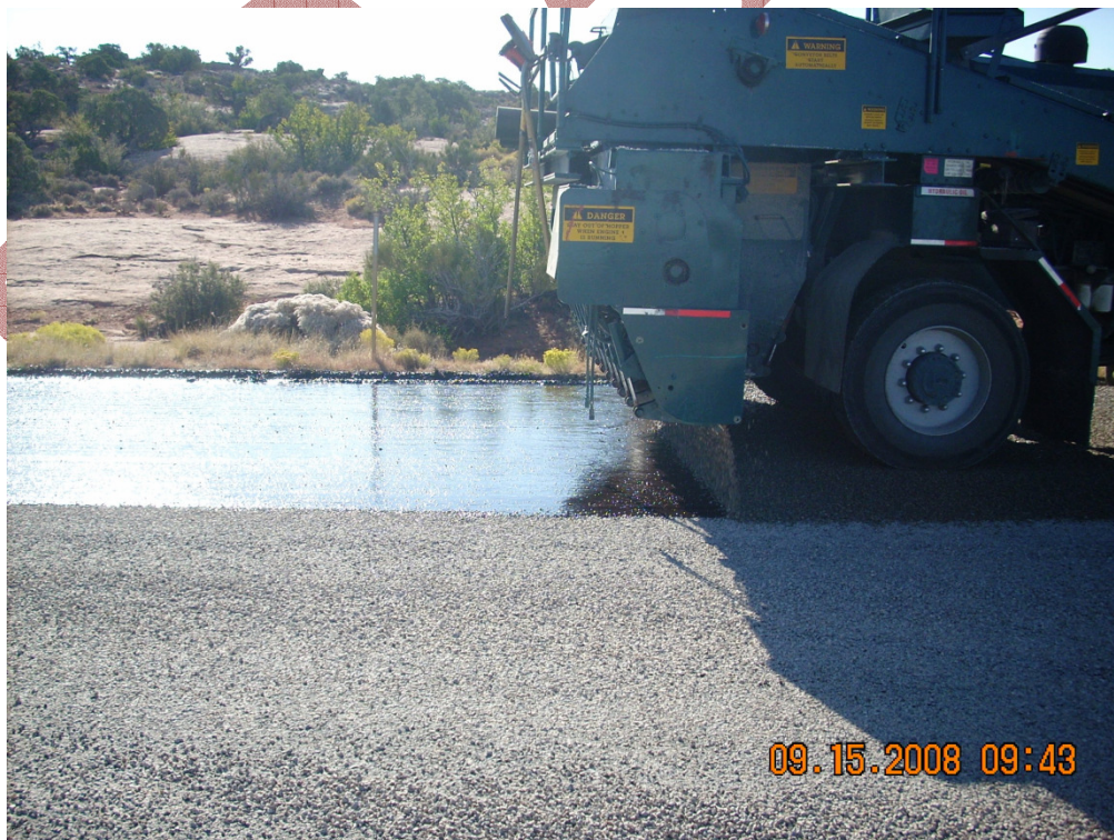
Figure 37: Utah Parks Project – Canyonlands NP Chip Seal Chip Application
