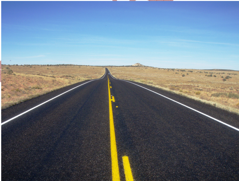
Figure 39: Utah Parks Project – Canyonlands NP Finished Chip Seal After Fog and Striping
