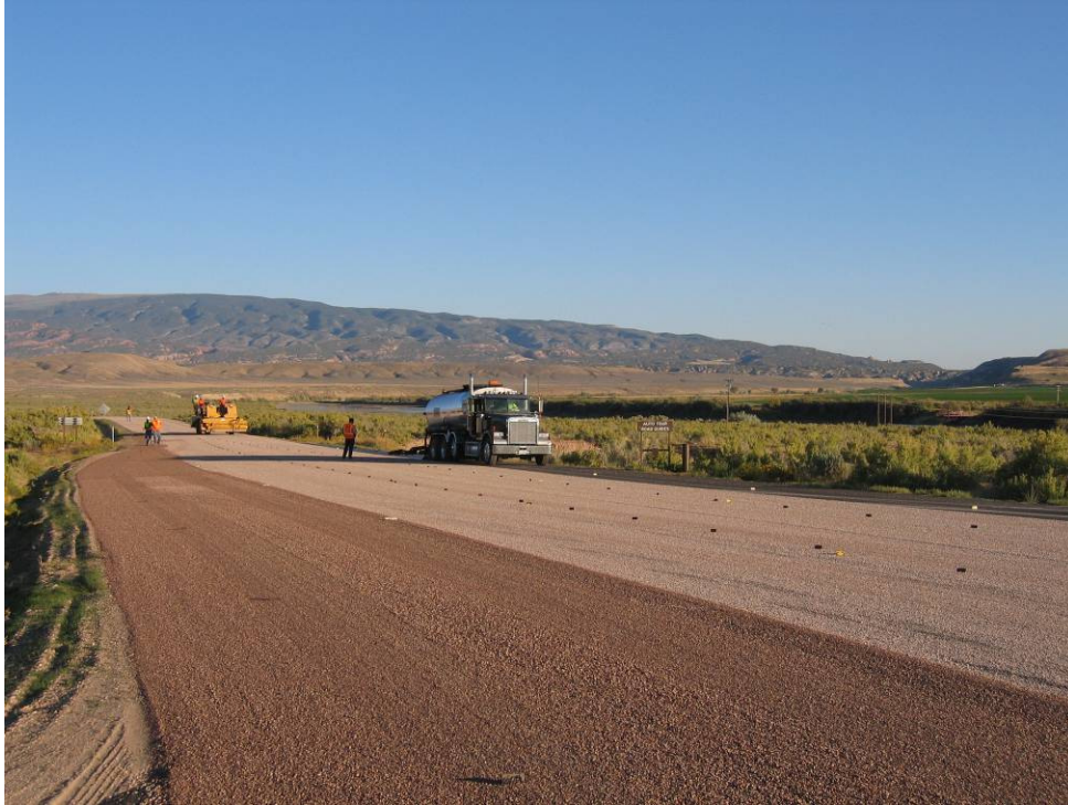
Figure 30: Dinosaur Project - Pay Station Chipsealing
