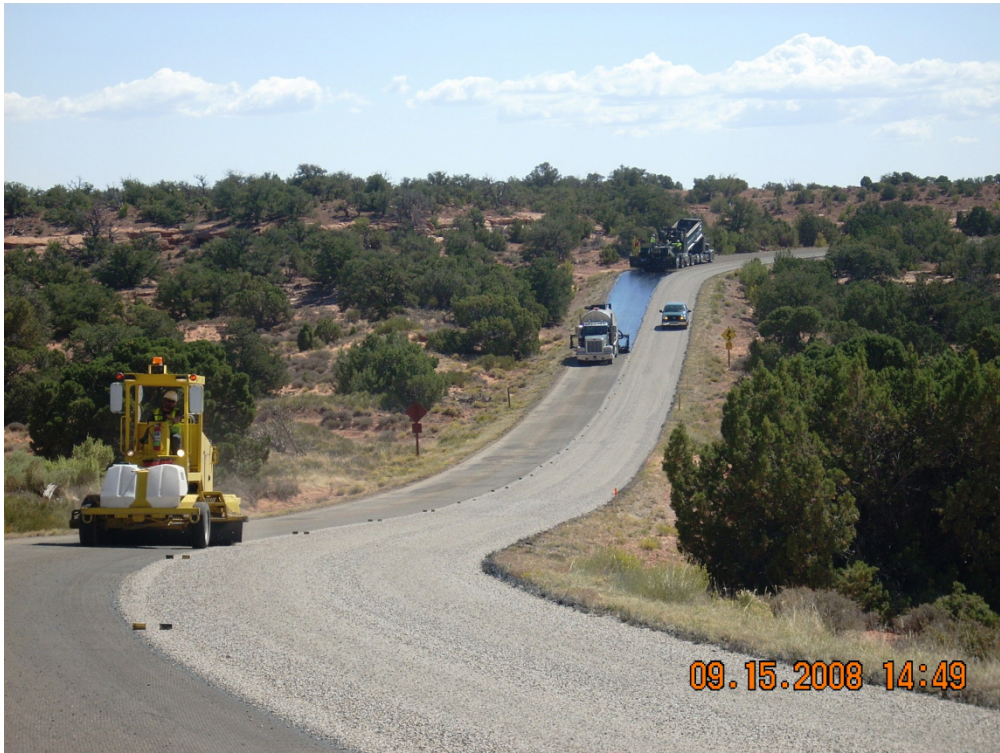
Figure 38: Utah Parks Project – Canyonlands NP Chip Seal Construction
