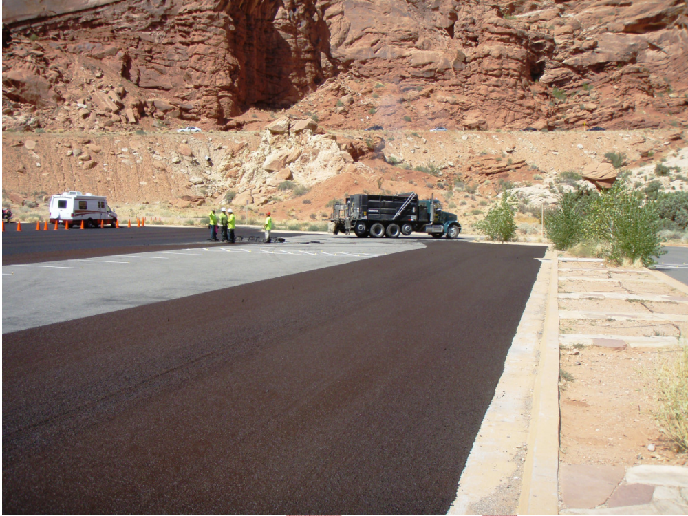
Figure 34: Utah Parks Project – Microsurfacing at Arches National Park
