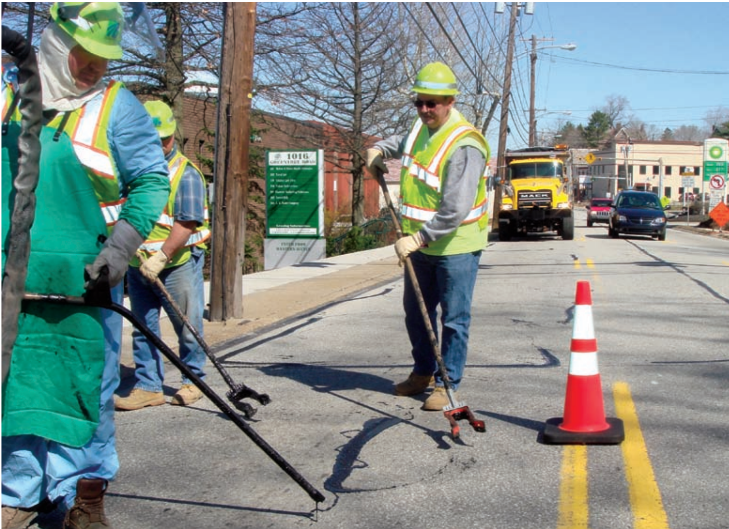
PennDOT workers engage in crack sealing to keep moisture from penetrating beneath the road surface. In Pennsylvania, which has a vigorous freeze-thaw cycle each winter, keeping moisture out of the area beneath road surfaces is a critical maintenance step.
