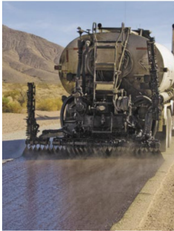
Figure 42: Death Valley Project – Chip Seal Emulsion Application
