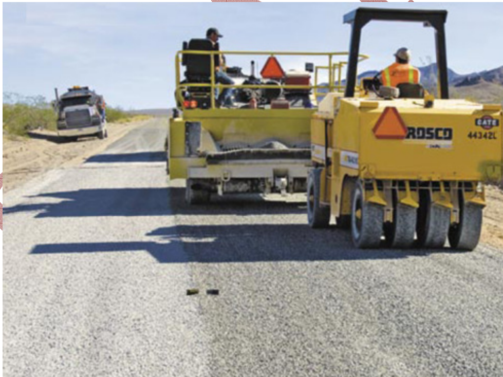
Figure 45: Death Valley Project – Rolling the Chip Seal
