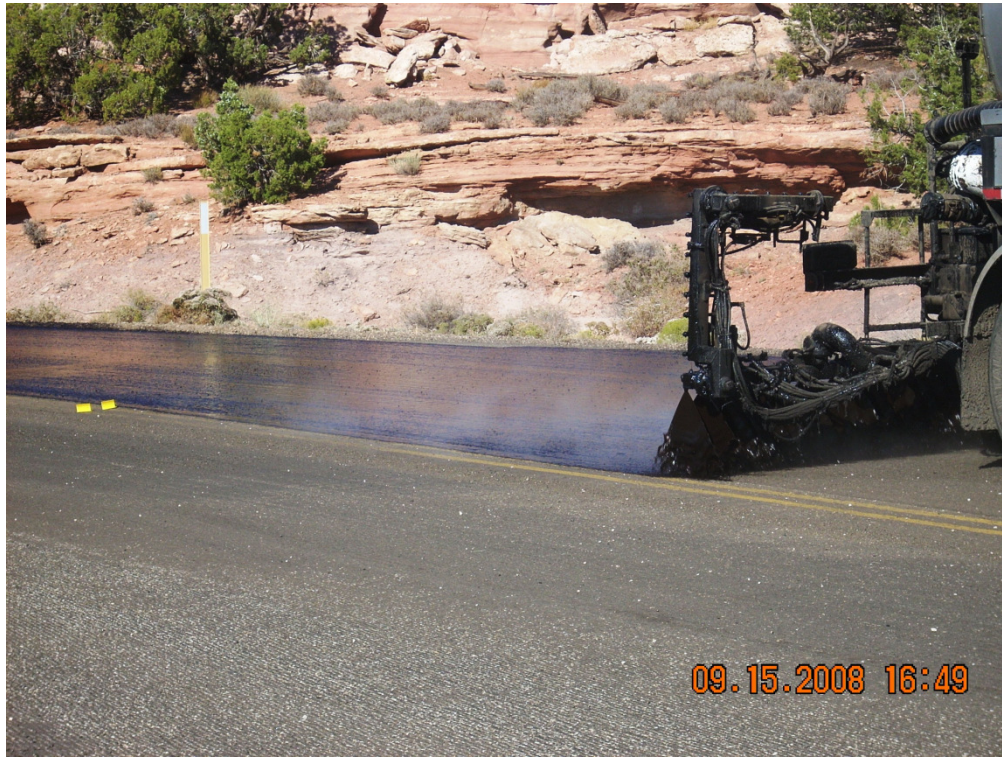
Figure 36: Utah Parks Project – Canyonlands NP Chip Seal Emulsion Application
