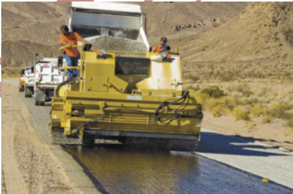
Figure 43: Death Valley Project – Chip Seal Aggregate Application
