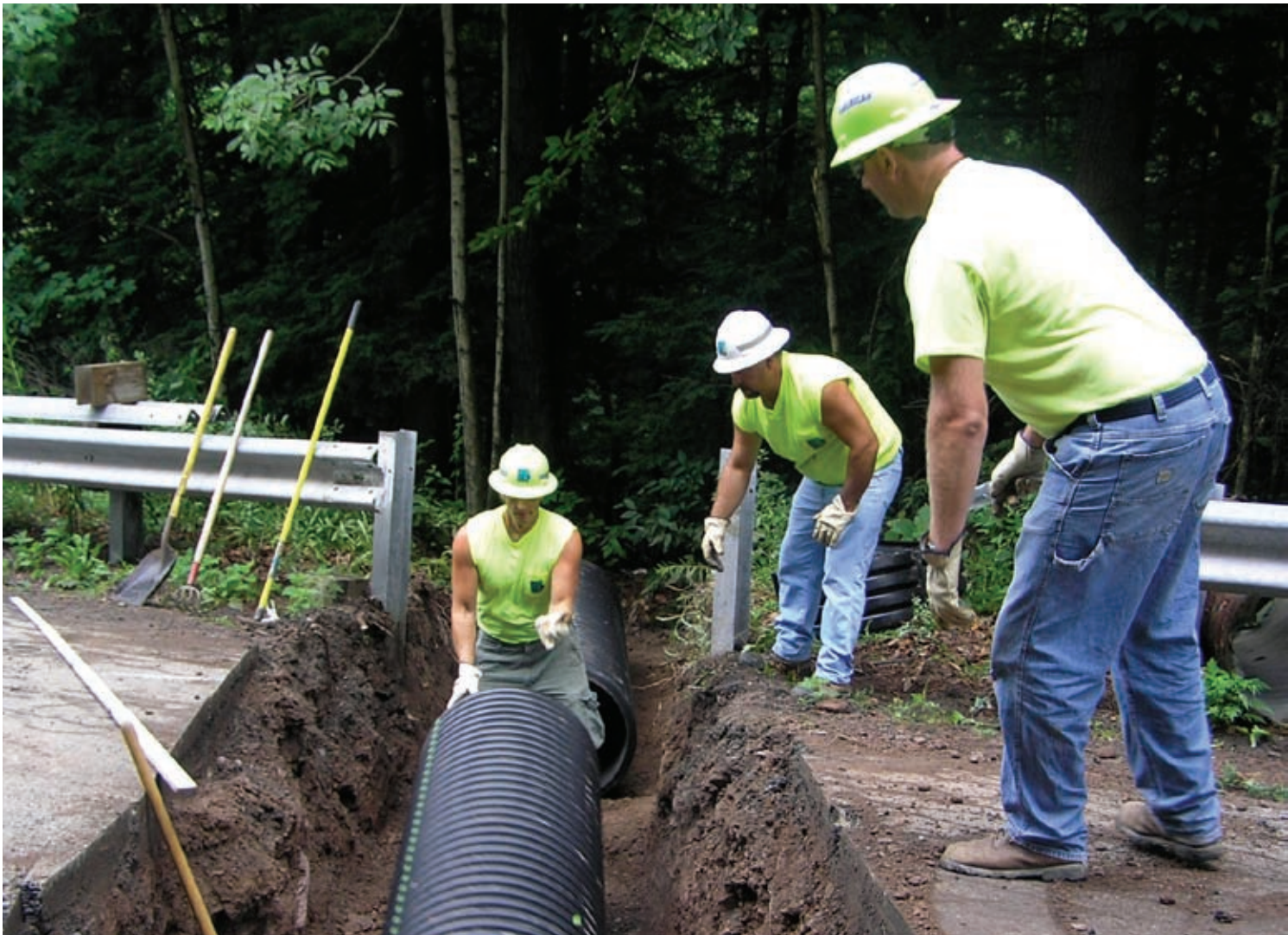
PennDOT workers lay replacement drainage pipe as part of a road maintenance project. Proper drainage for streams that cross beneath roads is a critical maintenance step.
