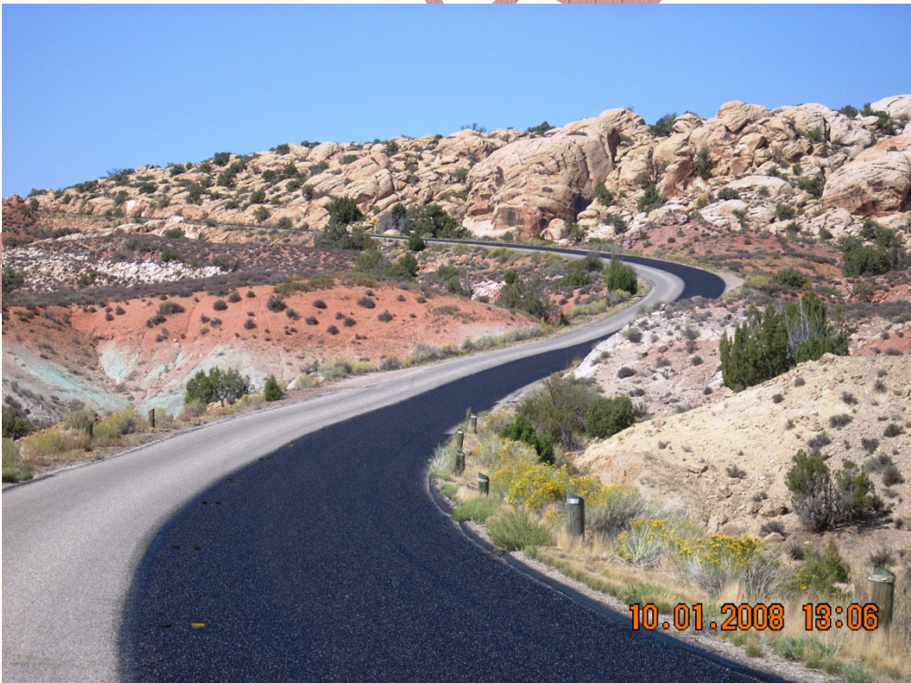
Figure 35: Utah Parks Project – Arches NP Partially Fogged
