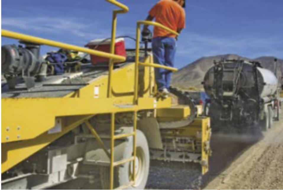
Figure 44: Death Valley Project – Chip Seal Construction
