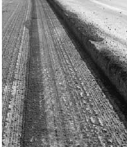
FIGURE 7 Milled HMA surface before overlay.
