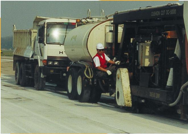
*Top: Diamond grinding under way at runway centerline
