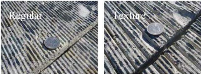
**Figure 5.** California I-280 conventional diamond grinding versus texture grinding<sup>6</sup>.
