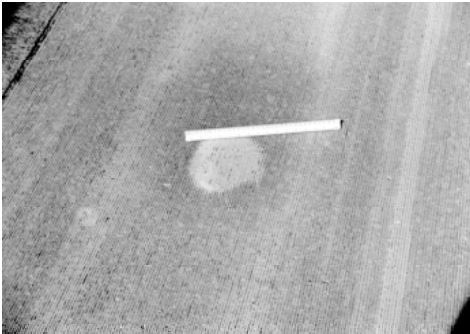
Figure 33. Sand-patch measurement for newly ground pavement.
