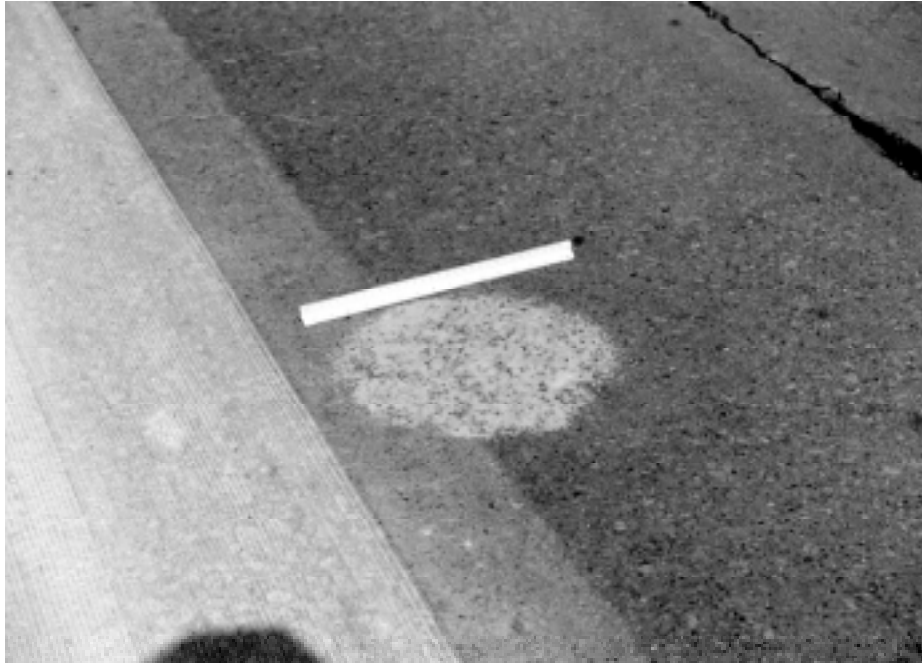
Figure 32. Sand-patch measurement for nonground pavement.
