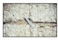
joint faces (see left). Even with recent advancements, incorporating greater numbers of machined teeth and a smoother drum, the carbide milling process falls short of the diamond grinding process. According to a Caltrans report, "Unless an agency is willing to accept badly spalled joints, the cold planer (rotomill) is
