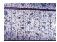
which is quieter than transverse textures. The longitudinal texture also enhances surface texture and skid resistance in polished pavements.
