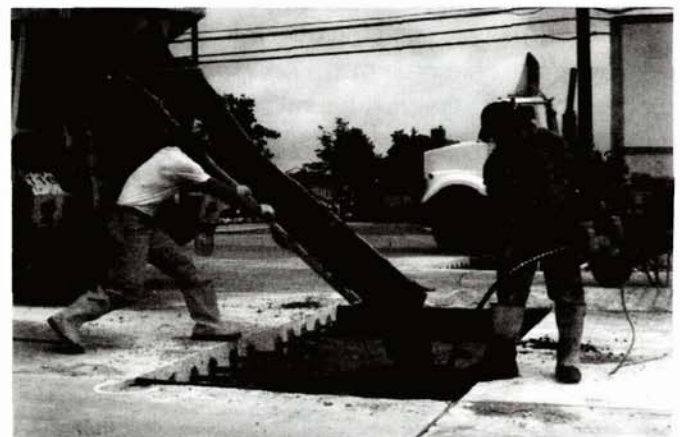
Figure 13. Chute operator and laborer filling a patch area and vibrating concrete in a suburban roadway patch.
