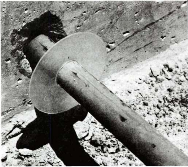
Figure 11. Grout-retention disk for holding in anchoring epoxy or mortar during dowel bar insertion.
