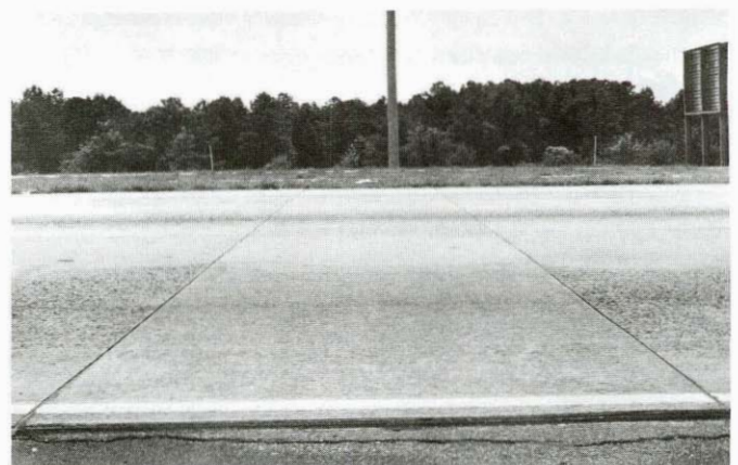
Figure 14. Completed patch with sealed joints.
