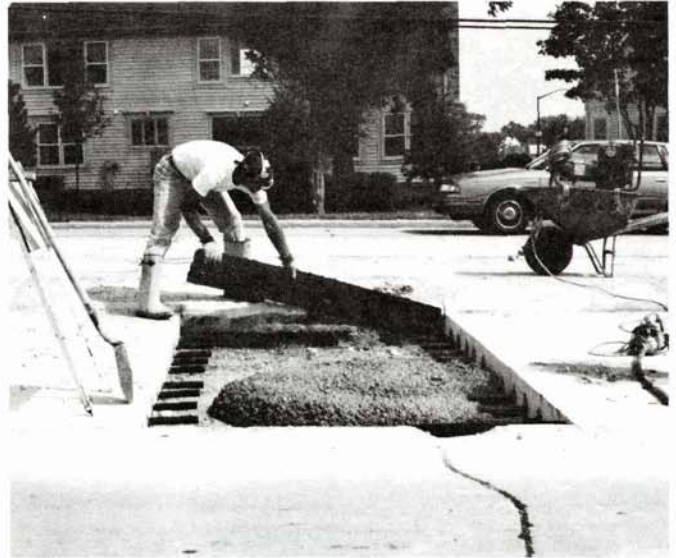
Figure 12. Worker placing bondbreaking board along longitudinal joint between patch and adjacent lane. Note: if the patch is longer than 4.5 m (15 ft) use tiebars or wigglebolts to tie the patch to the adjacent lane.
