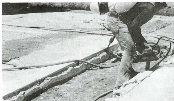
Figure 9. Chipping below vertical saw cut.
