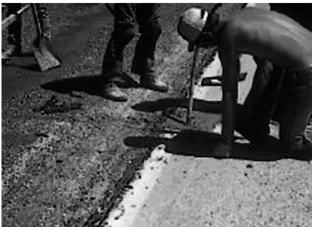
Figure 16. Consolidation of partial-depth repair material.
