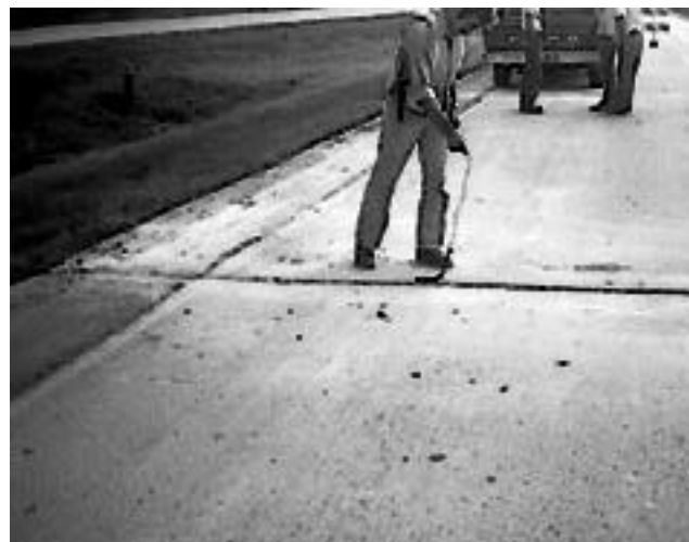
Figure 5. Sounding the pavement with a chain.
