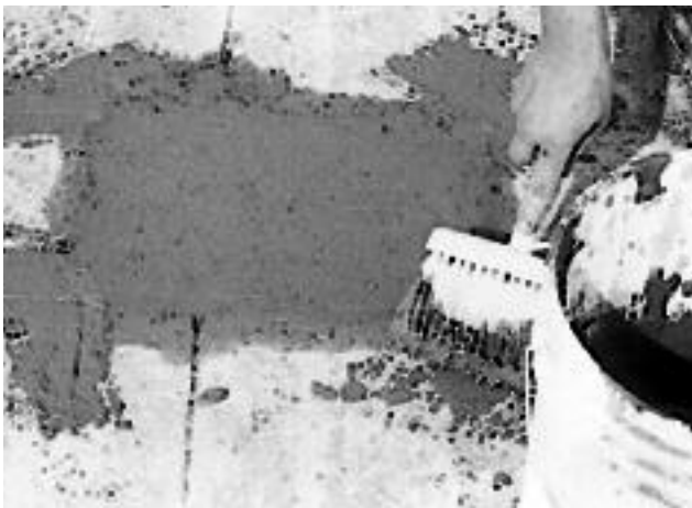
Figure 18. Sealing repair boundaries with cement-water grout.
