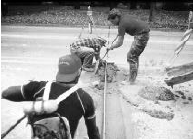
Figure 15. Placing partial-depth repair materials.
