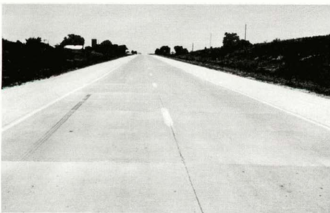
Pumping of fines on a rural highway. (Light areas near the transverse joints are the pumped fines.)
