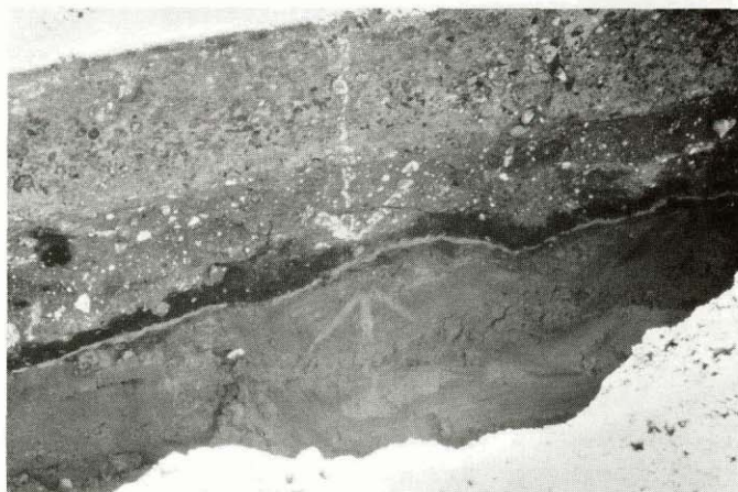
Successfully grouted void. Note the thin layer of grouting material between the slab and subbase.
