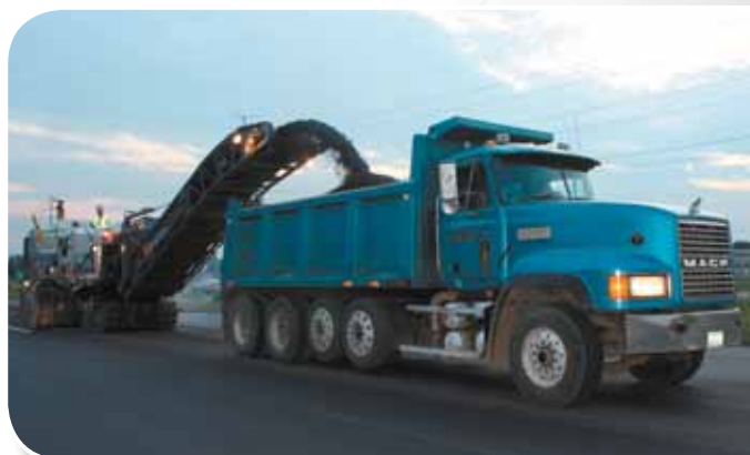
A Wirtgen W2200 cold mill conveys pavement millings into a Mack truck prior to placement of highly polymer modified asphalt on Minnesota TH100.
