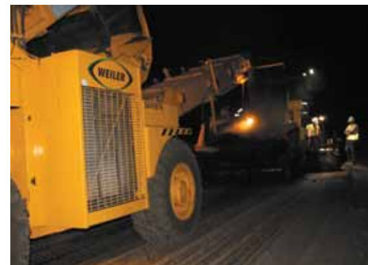
A Weiler E1250A materials transfer vehicle feeds HiMA mix for I-5 thin overlay into Blaw Knox paver.
