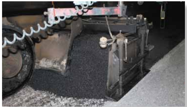
HiMA mix at approximately 290 degrees Fahrenheit is laid out by paver, exhibiting no viscosity problems.
