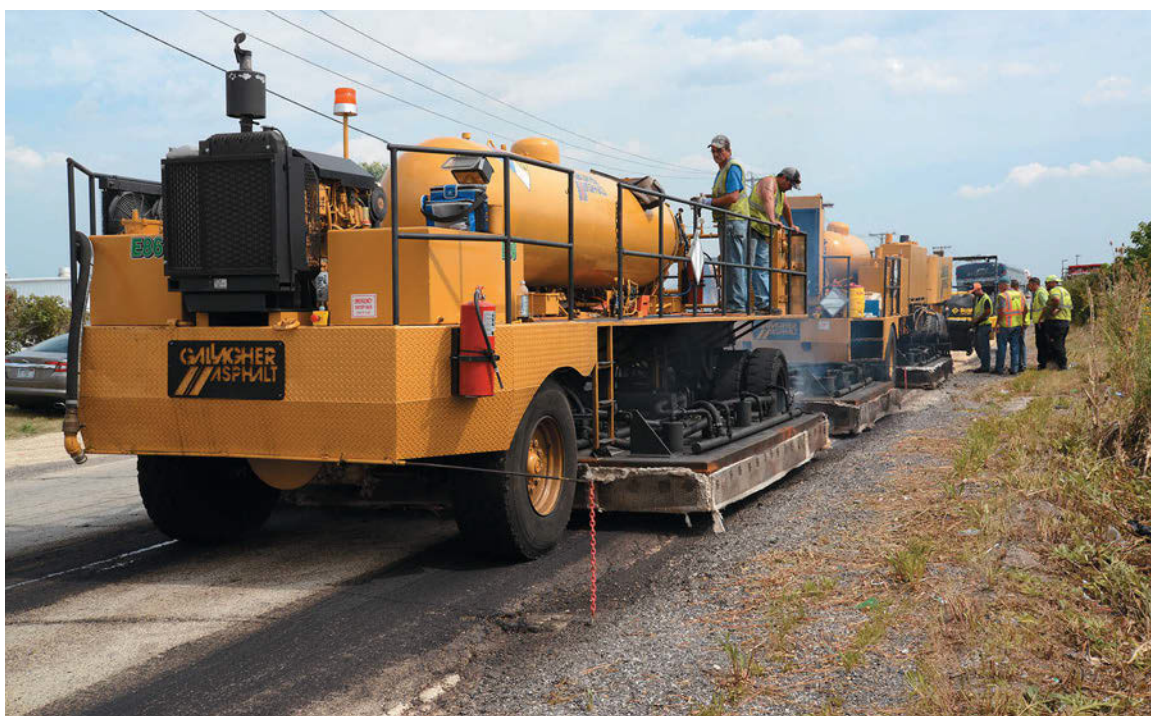
While delegates watch, Gallagher Asphalt demonstrates hot in-place recycling method
