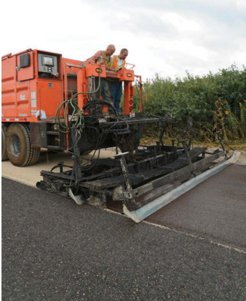
HIR section gets micro surfacing overlay placed by Rock Solid Stabilization & Reclamation, using Bergkamp mobile equipment
