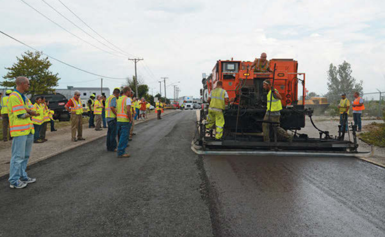
In one pass, contractor Dunn Company cold in-place recycles pavement using Wirtgen 3800 CR, grinding and mixing with engineered asphalt emulsion from Asphalt Materials, Inc. (tanker at left off image), and placing cold mix in hopper of Vögele Vision 5100-2 paver
