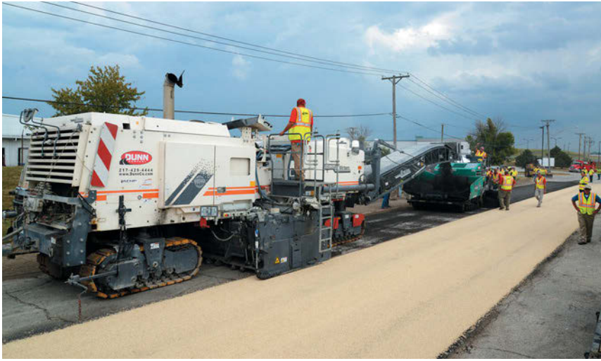
In one pass, contractor Dunn Company cold in-place recycles pavement using Wirtgen 3800 CR, grinding and mixing with engineered asphalt emulsion from Asphalt Materials, Inc. (tanker at left off image), and placing cold mix in hopper of Vögele Vision 5100-2 paver
