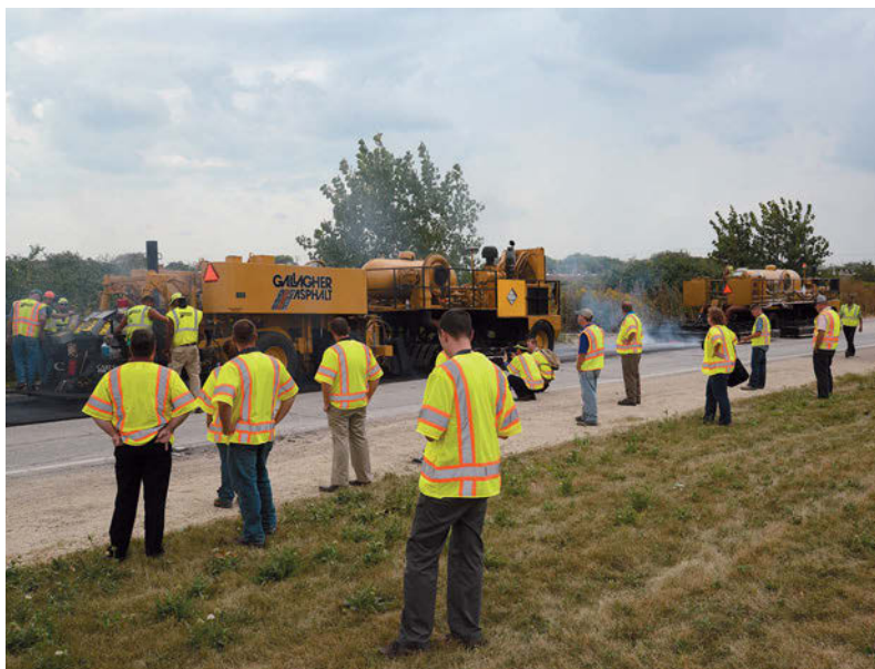
While delegates watch, Gallagher Asphalt demonstrates hot in-place recycling method
