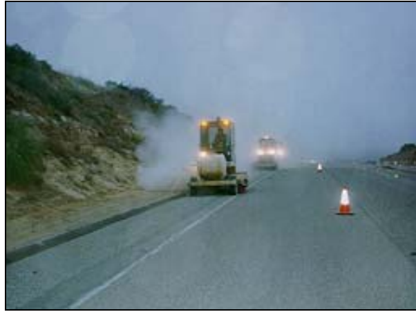
Figure 4-8 Brooming Process, Shown on a Shoulder Seal
