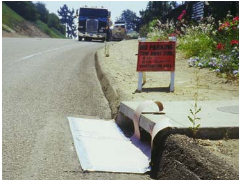
Figure 5-1 Protecting catch basin
