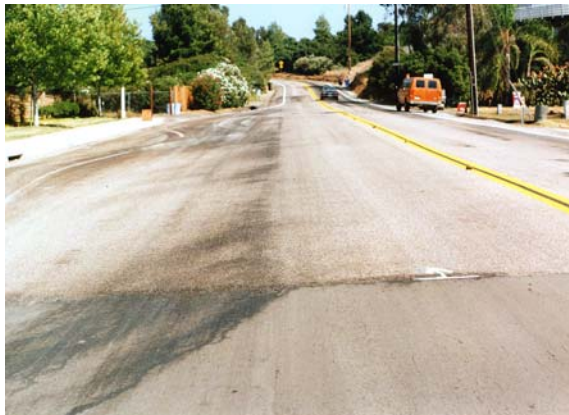
Figure 5-4 Chip Seal exposed to rain within 24-hours of placement
