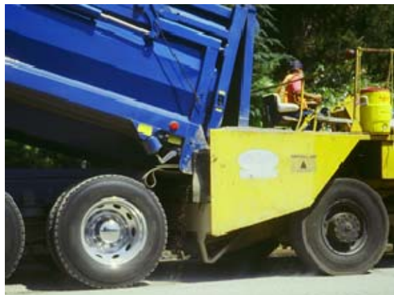
Figure 4-6 – Proper Connection
