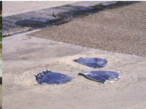
Figure 5-2 Protecting castings
