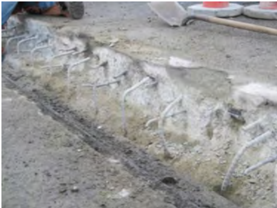
Photo No. 2 – Demolished Expansion Joint
