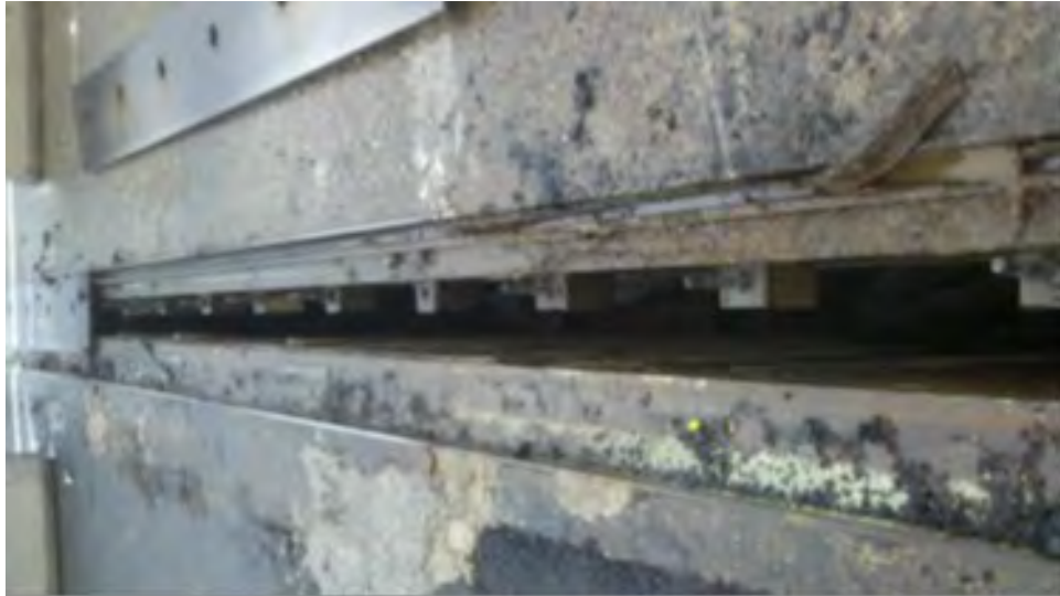
Photo No. 1 – Original Expansion Joint Prior to Demolition
