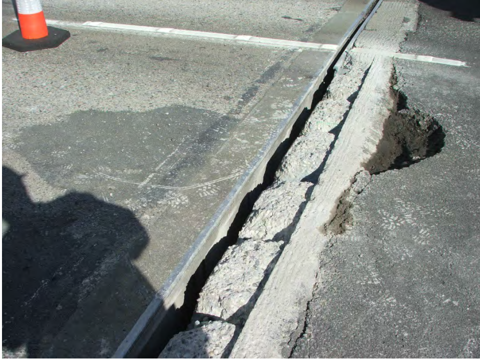
Photo No. 3 – Header After Steel Extrusion Was Removed
