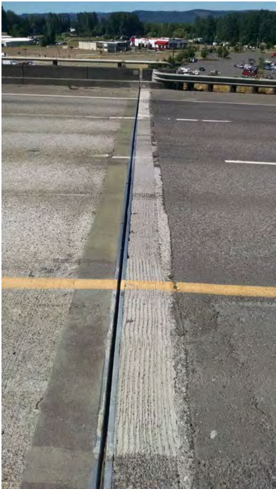
Photo No. 1 – North Abutment Expansion Joint
