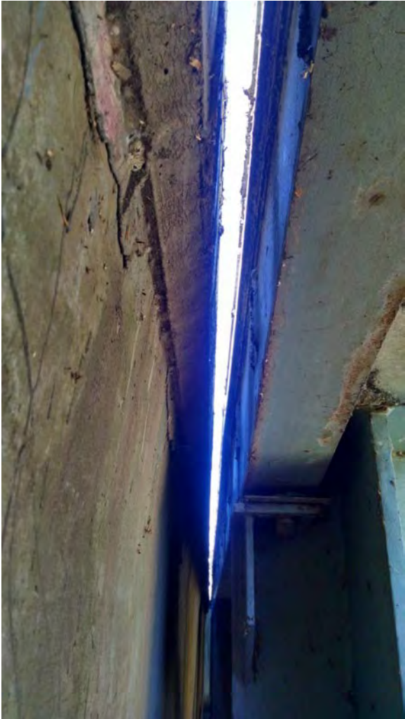
Photo No. 5 – South Abutment Strip Seal Expansion Joint From Below
