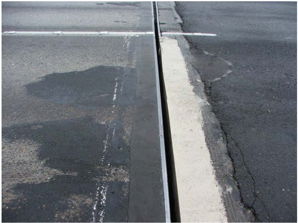
Photo No. 4 – Completed Repair
