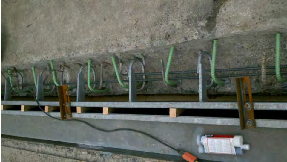
Photo No. 3 – New Steel Extrusions In Place Prior to Concrete Placement
