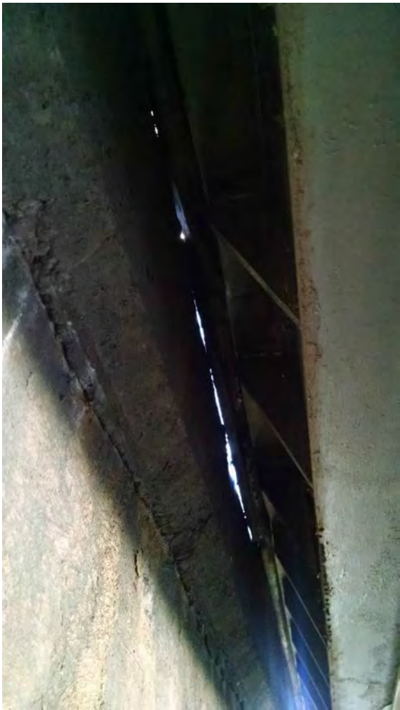
Photo No. 2 – North Abutment Expansion Joint From Below
