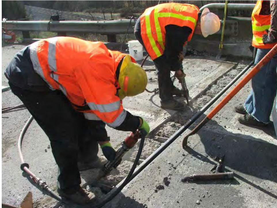
Photo No. 1 – WSDOT Maintenance Crew Removing Steel Extrusion From Abutment Side
