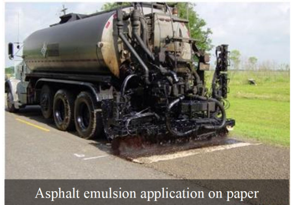
Figure 32: Creating a Perfect Transverse Joint on 15 lb/yd 2 Roofing Paper
