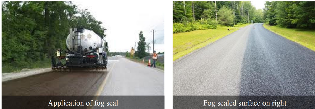
Figure 37: Application of an Emulsified Asphalt Fog Seal
