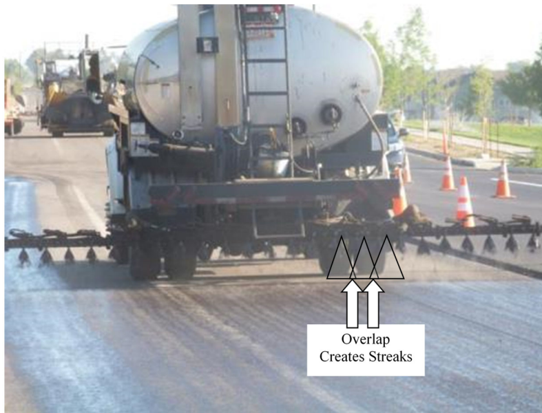
Figure 26: Photo of Spray Bar Set Too Low for No Overlap of Nozzles
