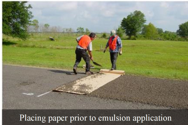
Figure 32: Creating a Perfect Transverse Joint on 15 lb/yd 2 Roofing Paper
