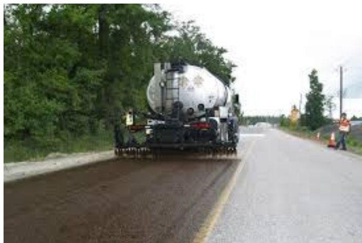
Figure 8: Fog Seal Application
