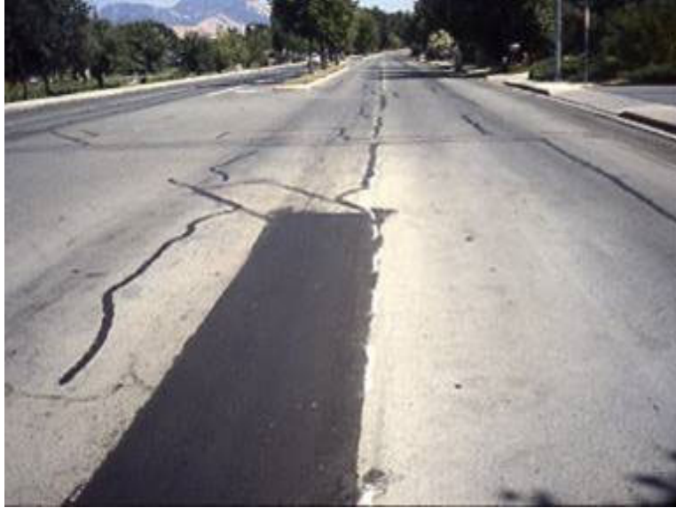
Figure 7: Crack Sealing and Patching
