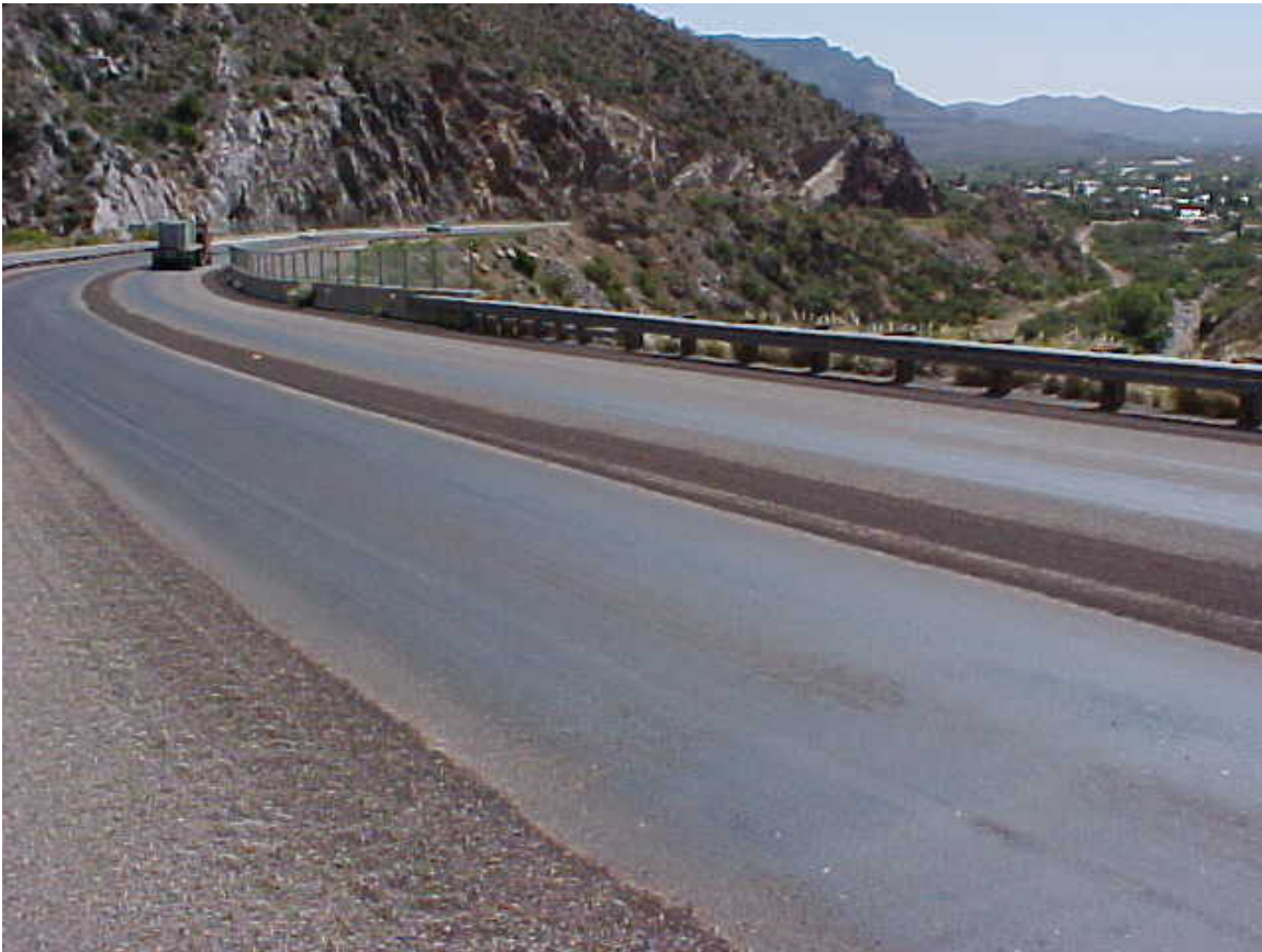
Figure 39: Aggregate Loss Problems
