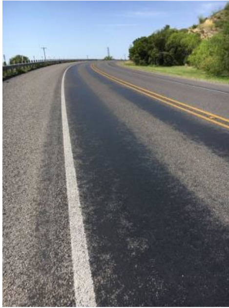
Figure 2: Flushed Pavement
