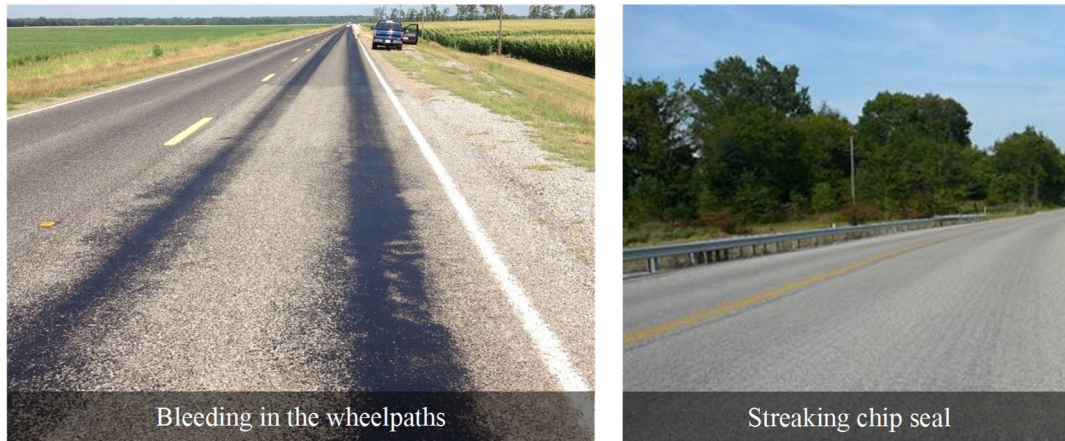
Figure 40: Typical Early Problems with Chip Seals
