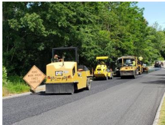
Figure 35: Rolling the Chip Seal
