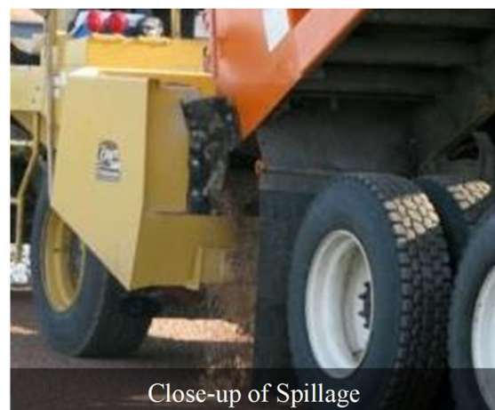
Figure 33: Aggregate Spillage Between the Truck and the Aggregate Spreader
