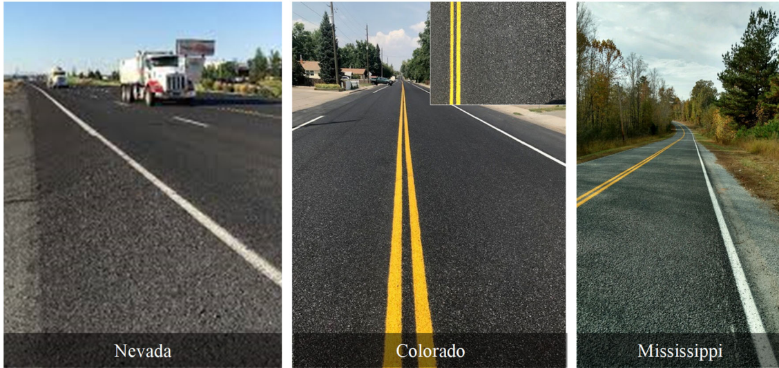
Figure 41: Good Completed Chip Seals Projects
