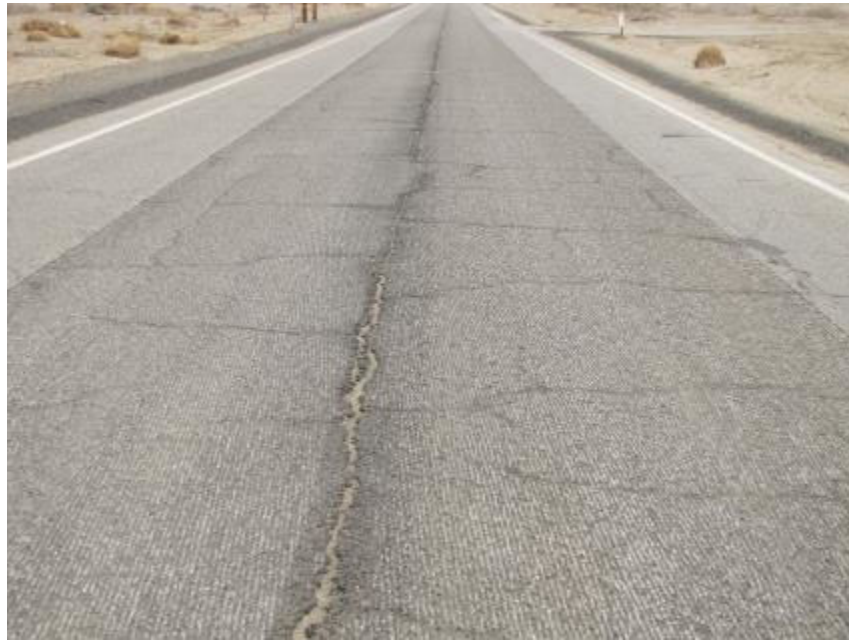
Figure 5: Micro Milled Surface
