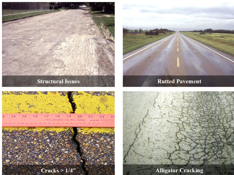
Figure 12: Examples of Pavements Not Acceptable for Chip Seals
