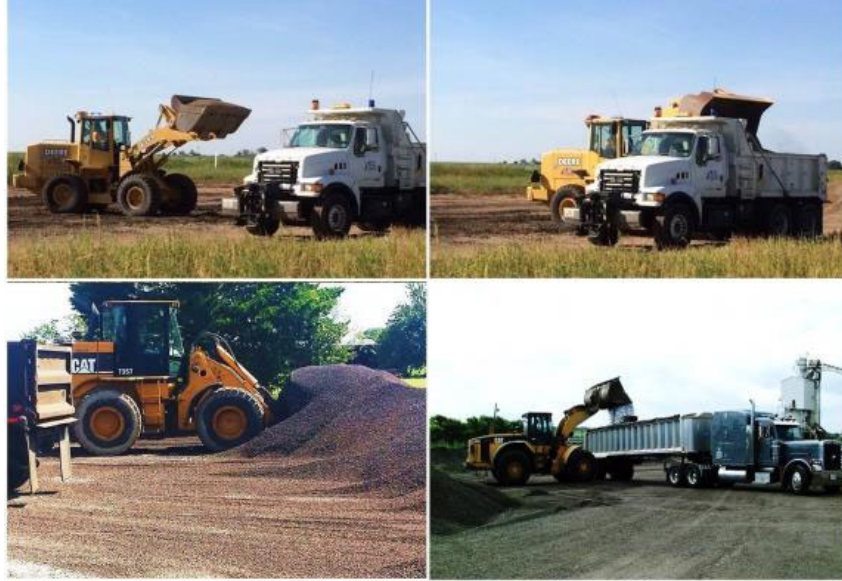
Figure 17: Loading from Stockpile onto Trucks
