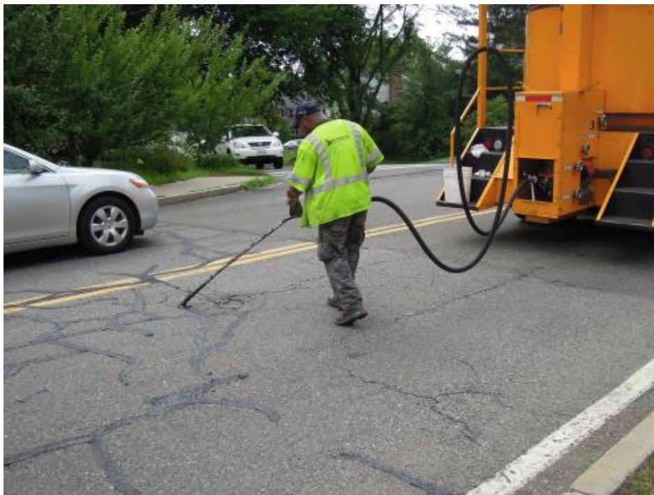
Figure 6: Crack Sealing
