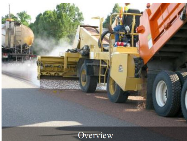
Figure 33: Aggregate Spillage Between the Truck and the Aggregate Spreader
