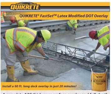
A complete 1/2" thick wear surface overlay and full-depth deck repairs can be made in one continuous application. QUIKRETE® FastSet™ Latex Modified DOT Overlay is a fiber reinforced, very low permeability, rapid-setting cementitious overlay material. Open to traffic in 3 hours.
