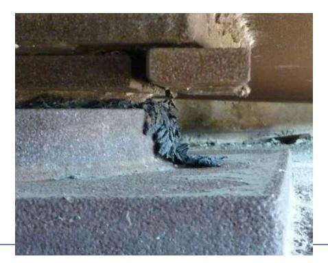
Number 1 issue is lack of funding to properly clean joint seals or finger joint troughs of debris on annual basis
