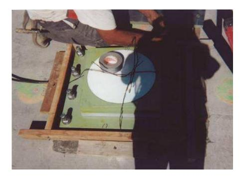
Properly position expansion bearings based on temperature and/or expected shrinkage and creep
