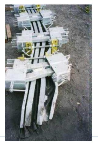
Avoid use of sledge hammer to position elastomeric bearings
