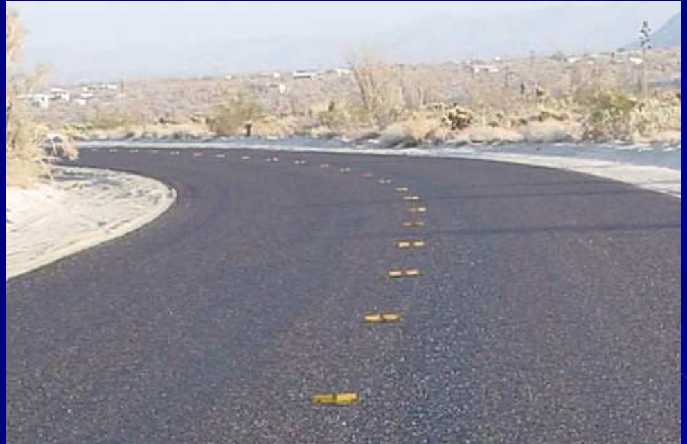
Remove Existing Pavement Markers and Place Temporary Pavement Markers
