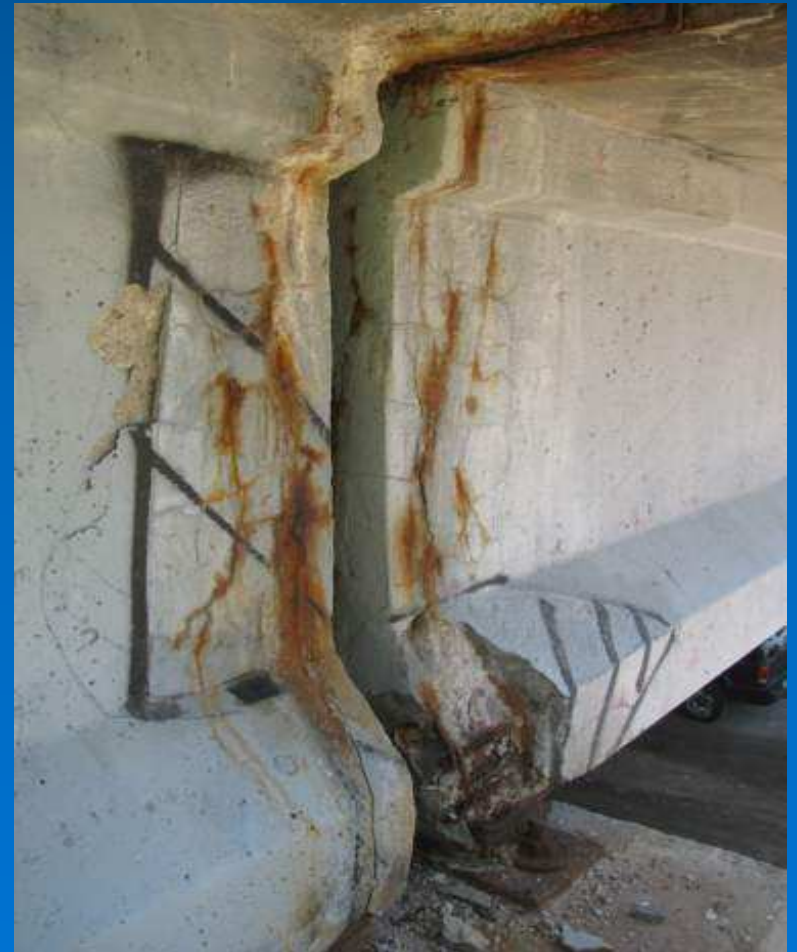
West Beams at Pier 3 - ECE
