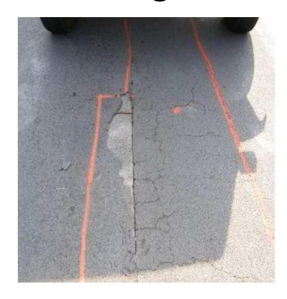
Premature failure of the Bridgemaster High Performance Polymer Slurry Overlay by Stirling Lloyd
