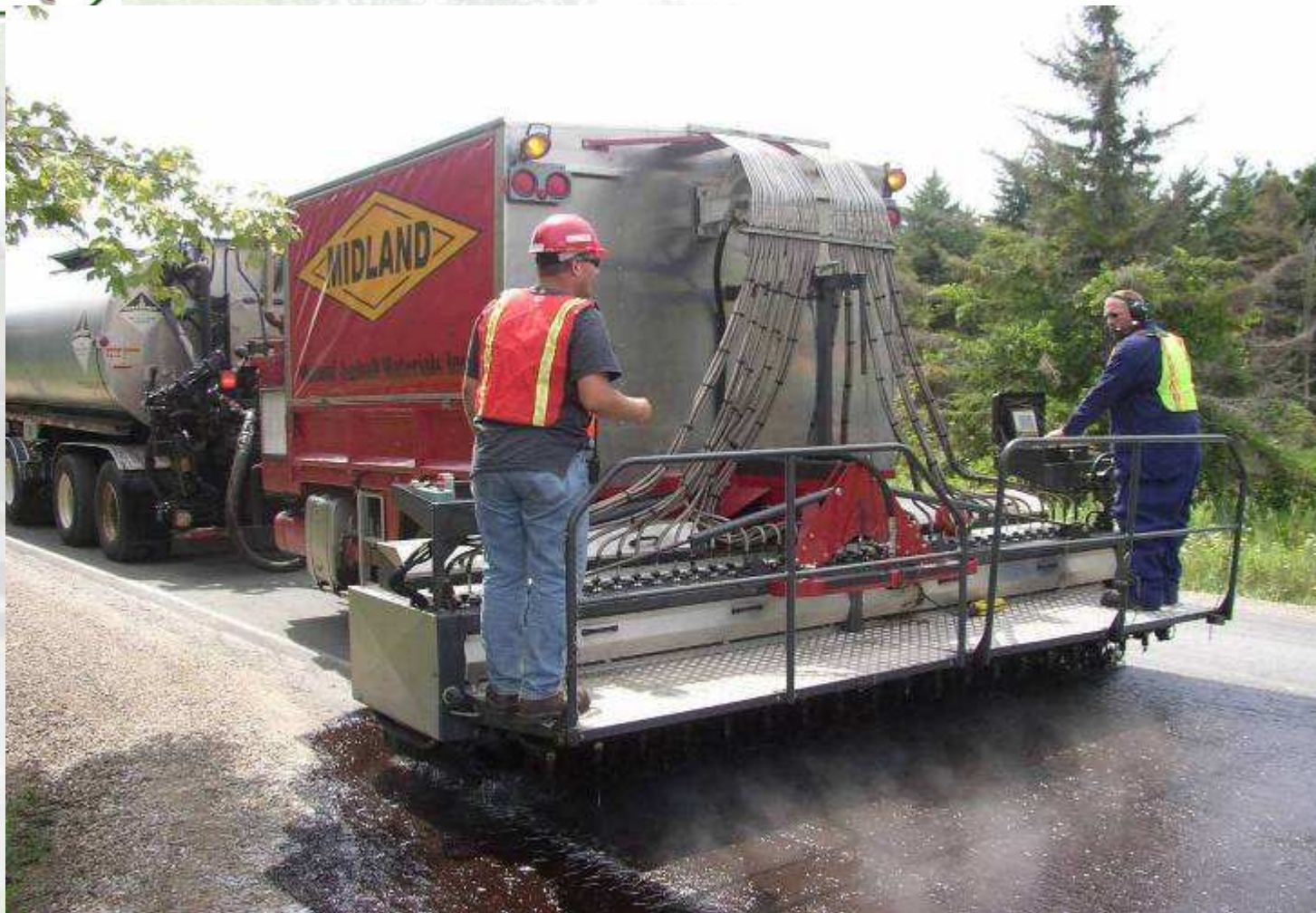
Trailer mounted 13 foot wide unit
