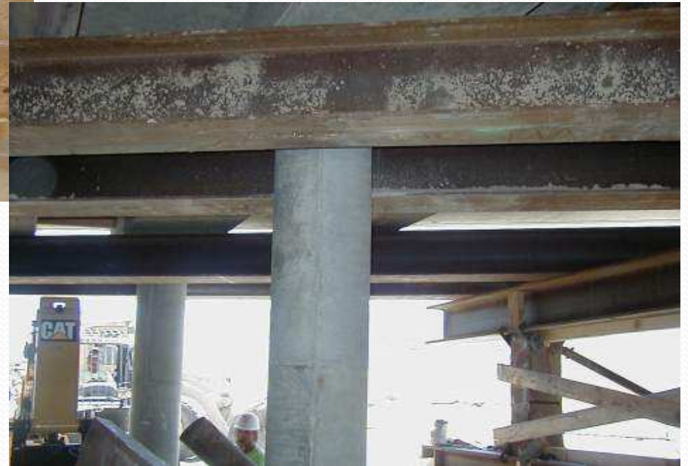
New Columns at Bent 5 of the Right Bridge
