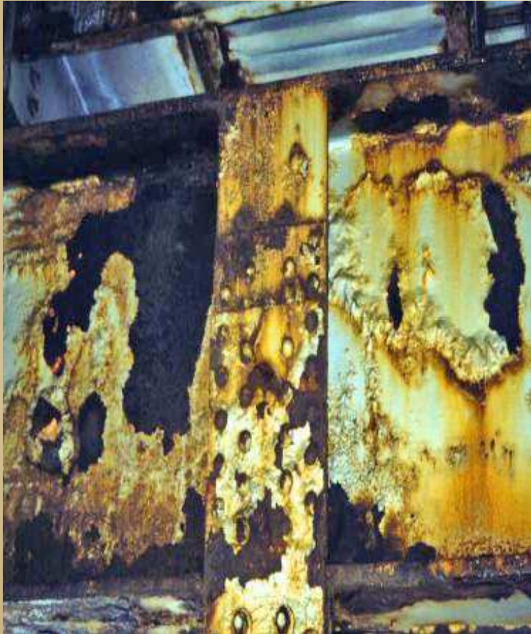
Rusting Steel – SSPC VIS2
