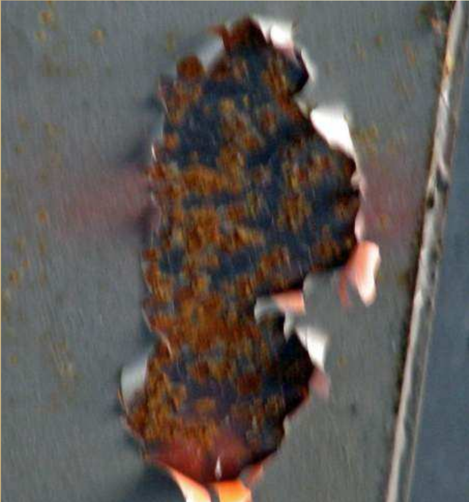
Disbonding/Peeling Paint
