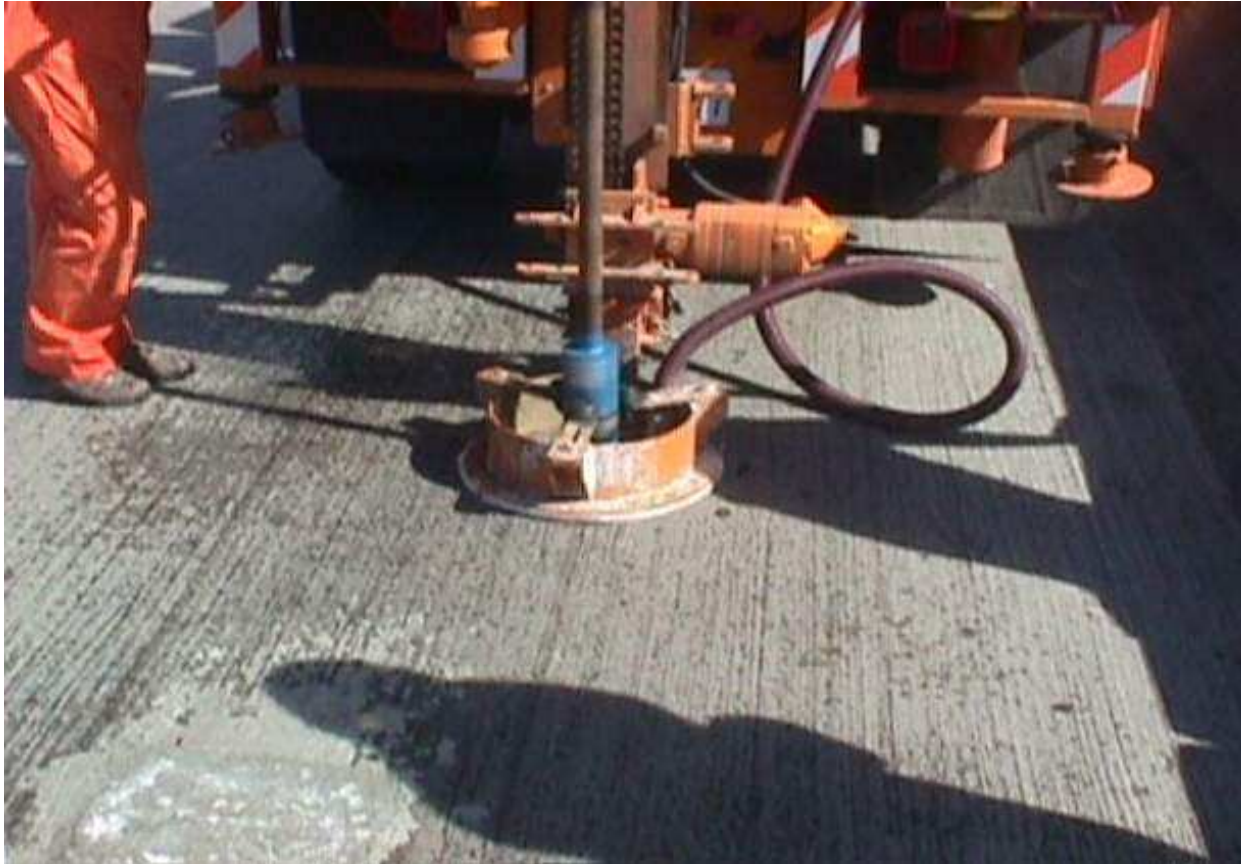
Concrete Core Operation
