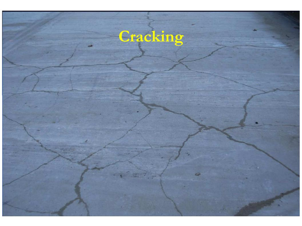
Ambient Air Temperature – 47 F – 50 F Humidity – avg. 18-20% Deck Temp. – 51 F Concrete Mix Temp. - 60 F Wind Speed - Sustained 10 mph, gusts to 25 +Concrete Mix Air Content – Avg. 5% 3 Hr. Cylinder Break – 4200 PSI
