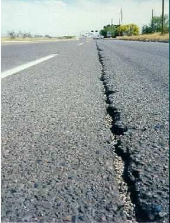
**Deteriorated Paving Joint** -Early in pavement life -Raveling -Accelerating deterioration -Requires maintenance -Shortened pavement life
