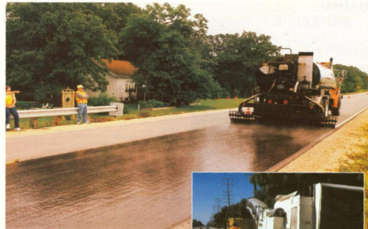
In Minnesota, a distributor truck sprays polymer-modified binder in advance of demonstration chip seal.
