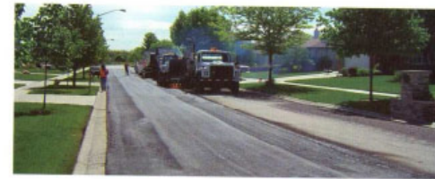
Gallagher Asphalt's crew starts recycling the second lane of a Tinley Park residential street. The two-block project was completed in one day last May and is part of a 350,000- to 400,000-cubic yard contract Gallagher has with the village this year.
