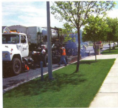
Gallagher's hot-in-place recycling train heats and scarifies old asphalt to a depth of 2 inches along the curb line. The train completes a 420-foot city block in less than an hour and residents have access to their driveways as soon as the train passes by.
