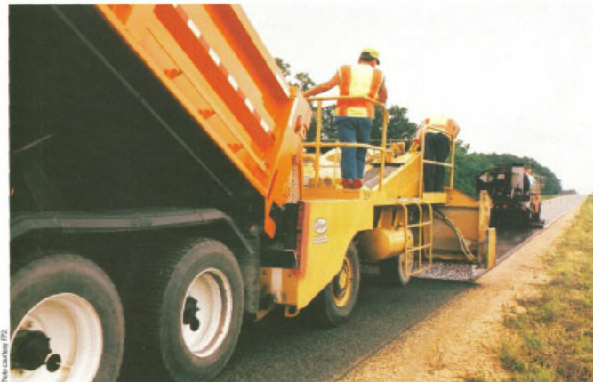
An Etnyre chip spreader places chips behind a distributor truck for a Minnesota chip seal demonstration.
