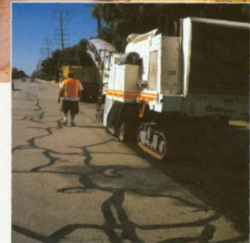
Beyond preservation, severely cracked asphalt friction course is milled in Ontario, California, by Lindy's Cold Planing, LaHabra.
